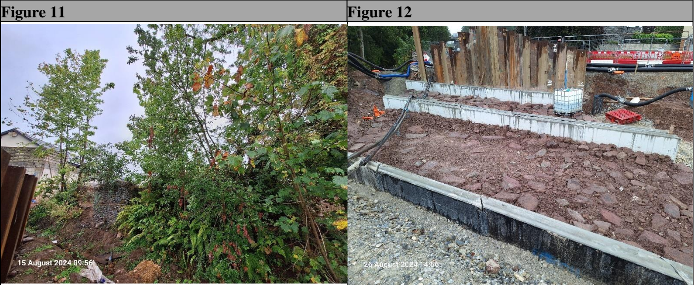
Caption 11 Caption 12 Trees surveyed prior to removal at Springmount. Flagstones placed in Brooklodge culvert and seeded with gravels.
