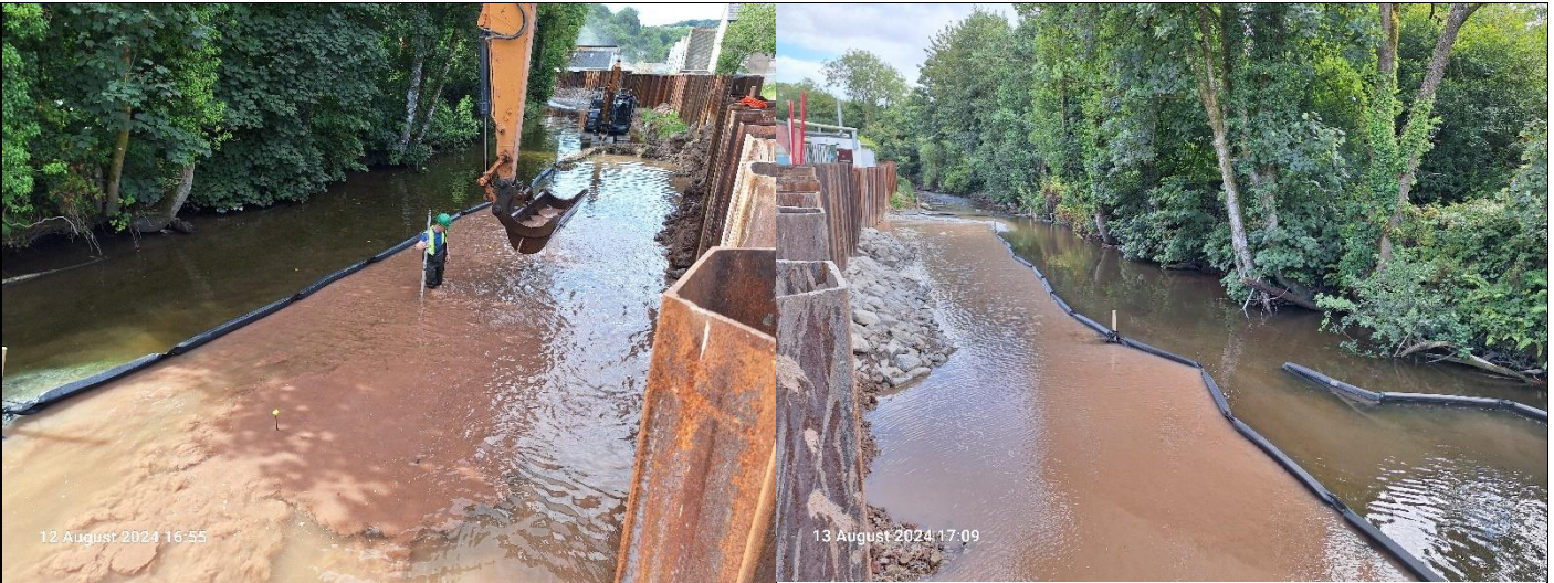
Caption 9 Caption 10 Rock armour works in Area 1, silt curtains installed parallel to works as well as diagonally downstream of works. Gravel checkdam installed at the lower extent of works to aid in the containment of silt.
