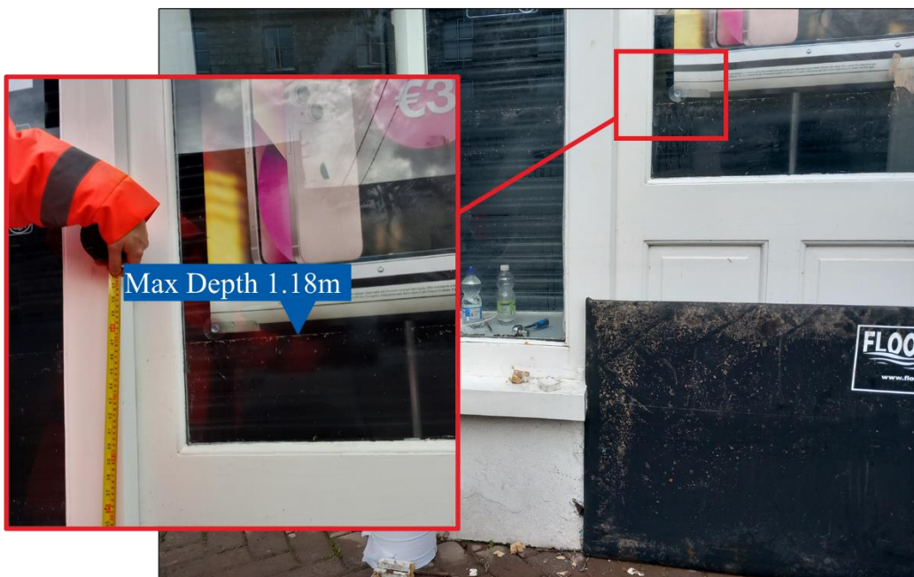
Figure 73: Wrack Mark at Three Shop
