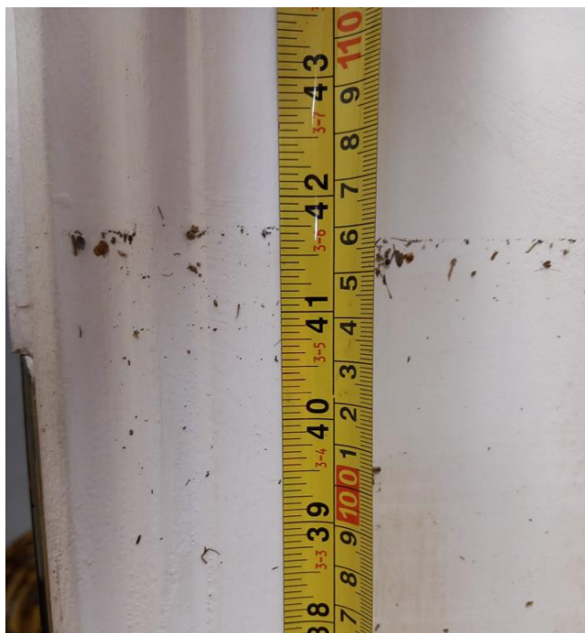
Figure 88: Wrack Mark at Water Rock House
