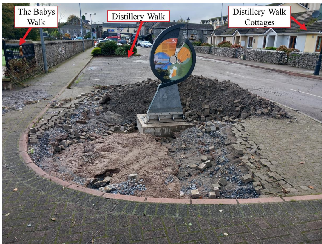
Figure 75: Scour Damage at Distillery Walk
