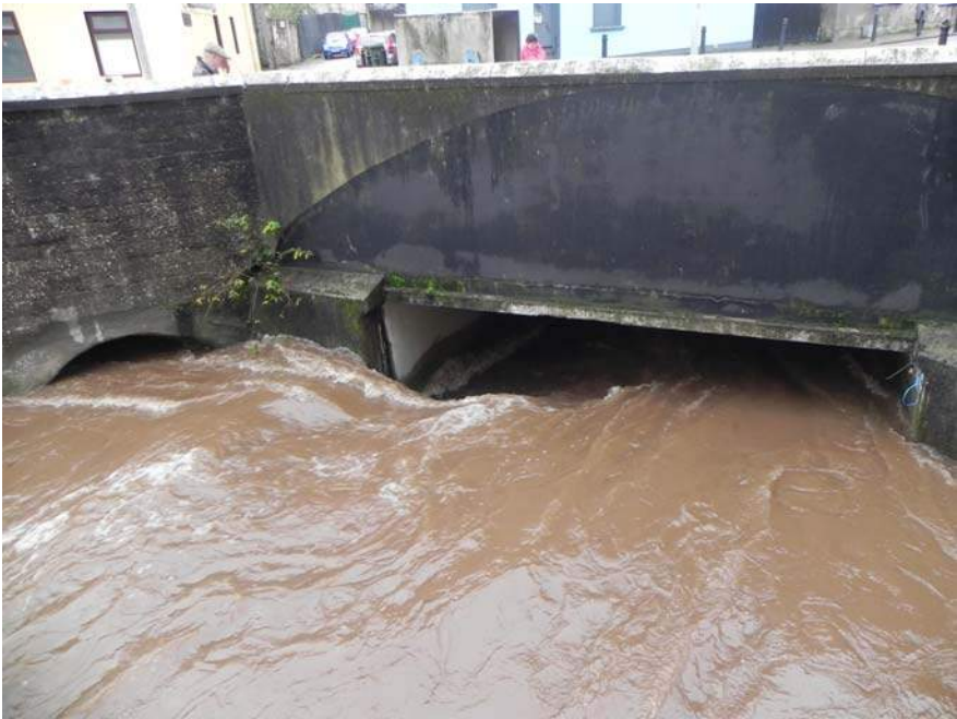
Fig 74: Standing wave at left side of culvert Channel
