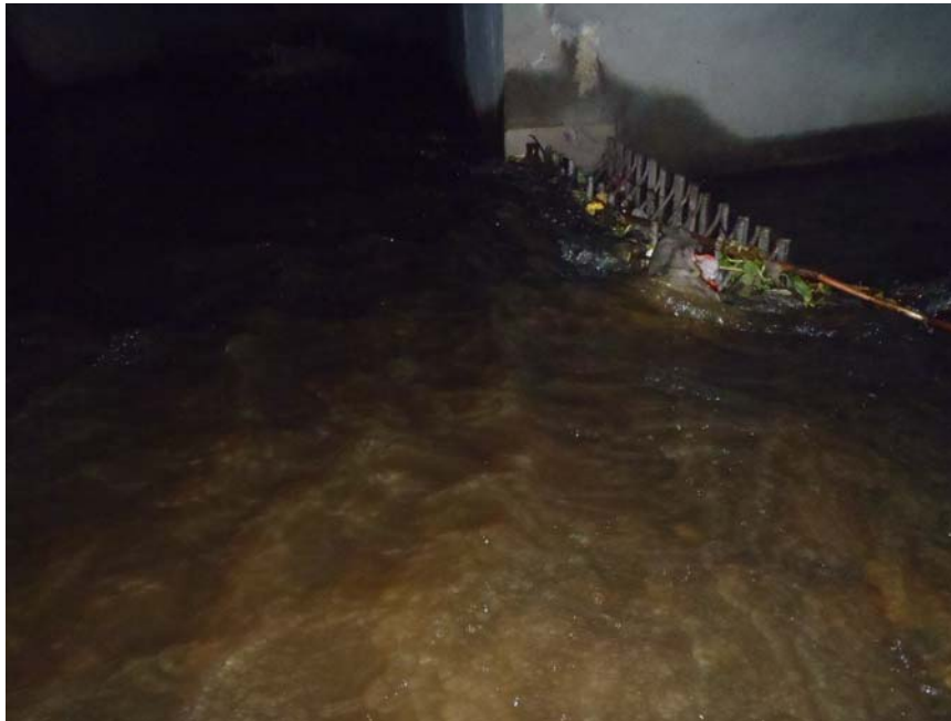
Fig 53: fouling on reinforcement structure in October:
