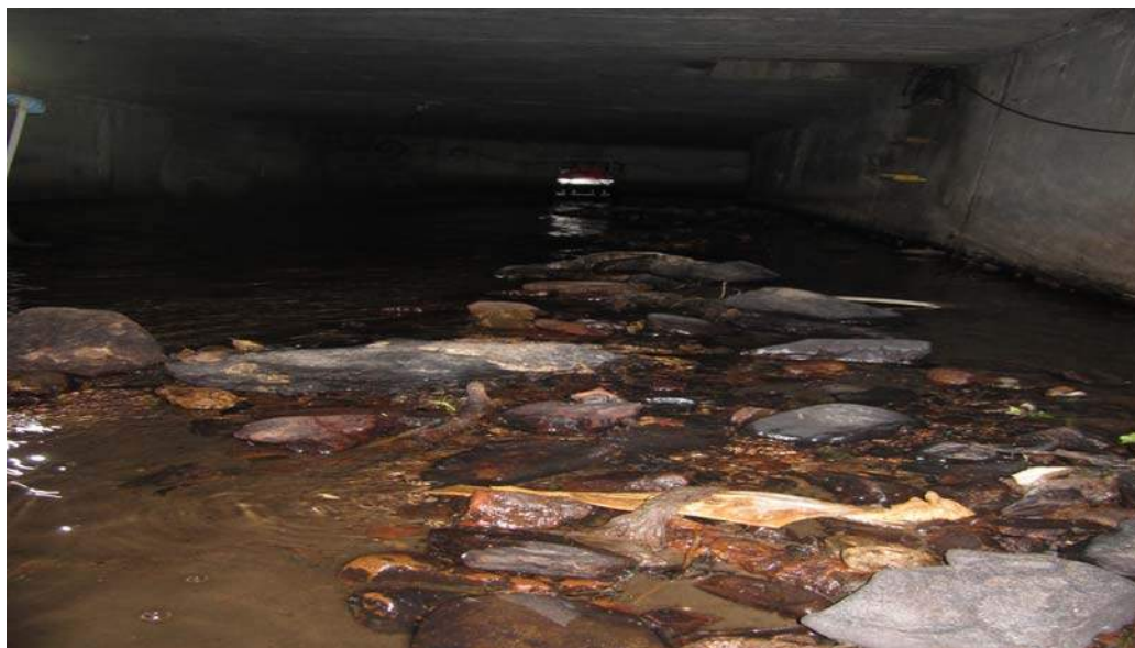
Fig 40: Stone accumulation in cross section at bifurcation during low levels:
