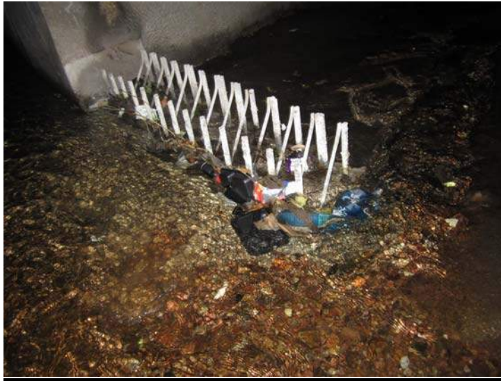
Fig 45: Reinforcement structure left after wall removed
