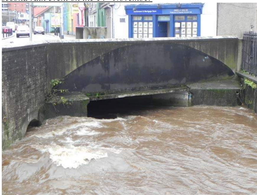
Fig 73: High Flow at the Culvert Entrance at Blackpool Church the morning after second rain event on the 14 th November
