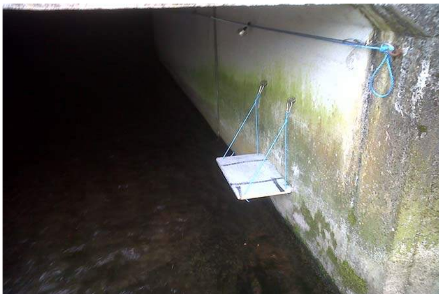
Fig 67: Standby man post with communications bell and safety line at Blackpool church culvert entrance
