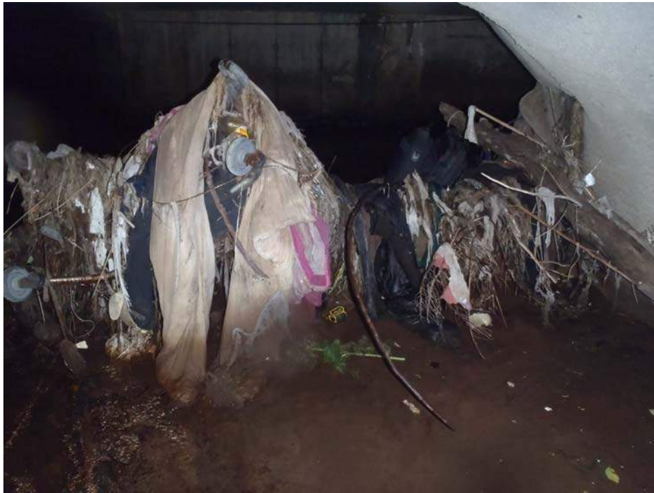
Fig 37: Debris trapped on wall at entrance to old brewery culvert ( FM2) looking back from FM2 probe.
