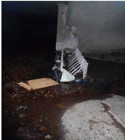
Fig 45: Reinforcement structure left after wall removed
