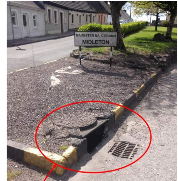
Manhole covering karst conduit
