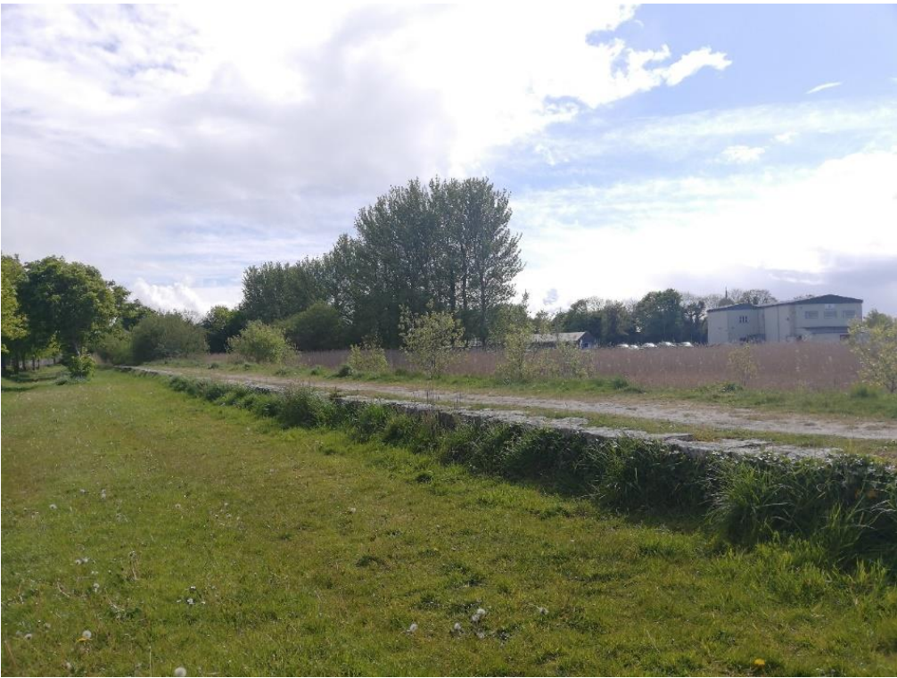
Figure 1.4.6 Dyke road embankment
