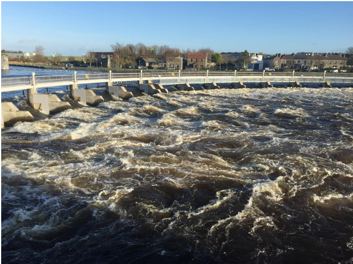
Plate 1 View of Salmon Weir taken on the 11 December 2015 during flood conditions with all gates opened
