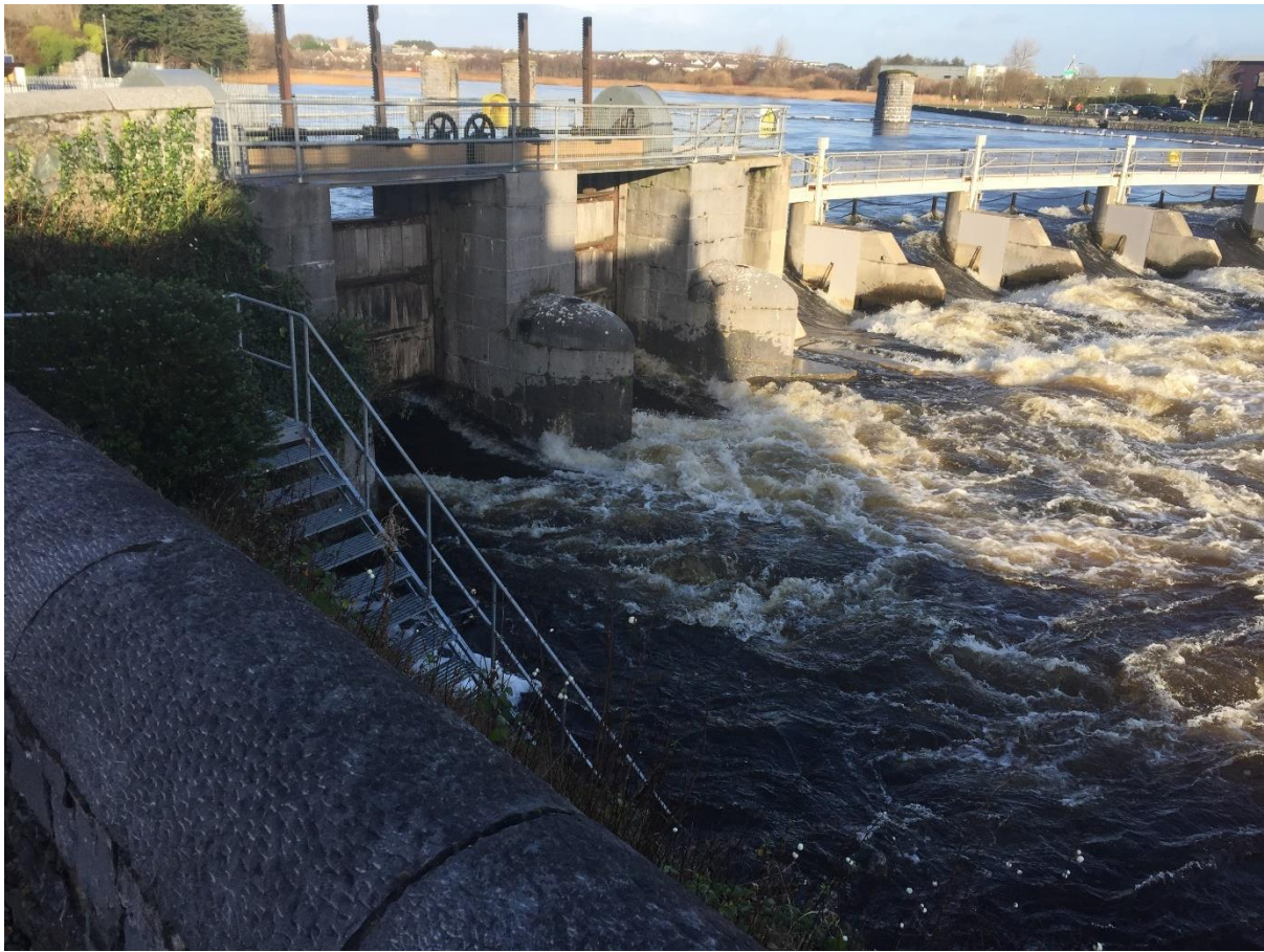
Plate 2 View of the two timber lift/drop gates taking during flood flows on the 11 th December 2015
