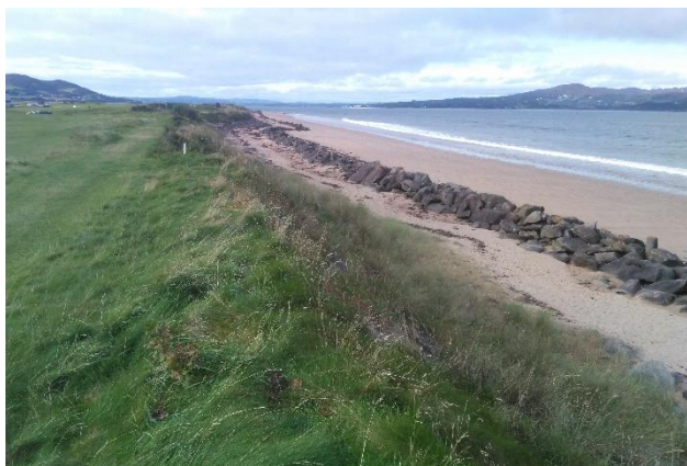
Rock Armour Protection, Buncrana Beach October 2021
