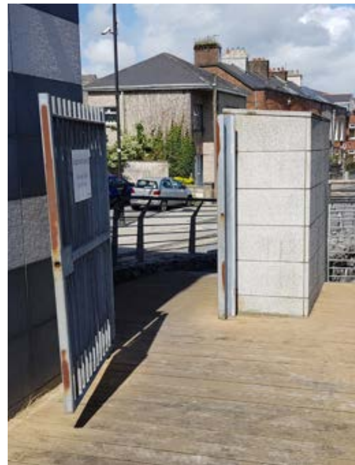
Northern boardwalk landing as existing
