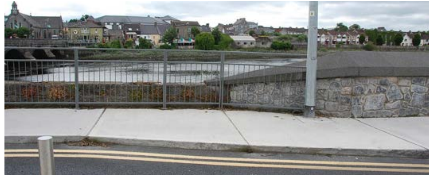
Photomontage showing the exposed concrete sections painted a darker shade of grey.
