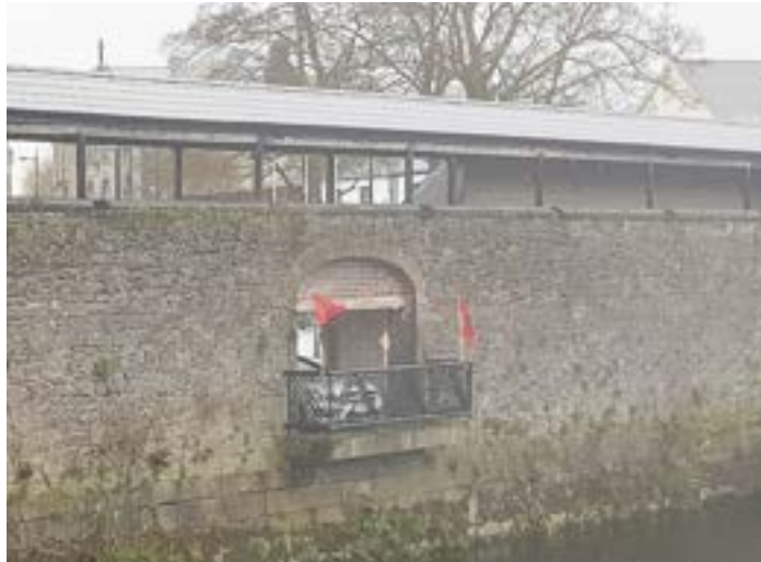
Railing to be replaced with glass panels across opening.
