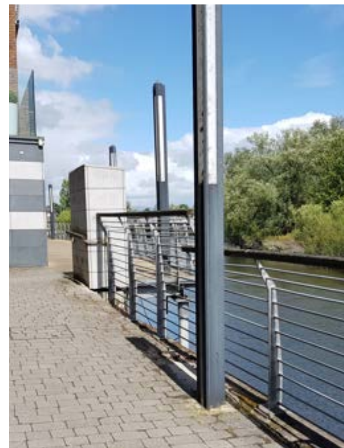
Existing railing to be replaced with new wall.
