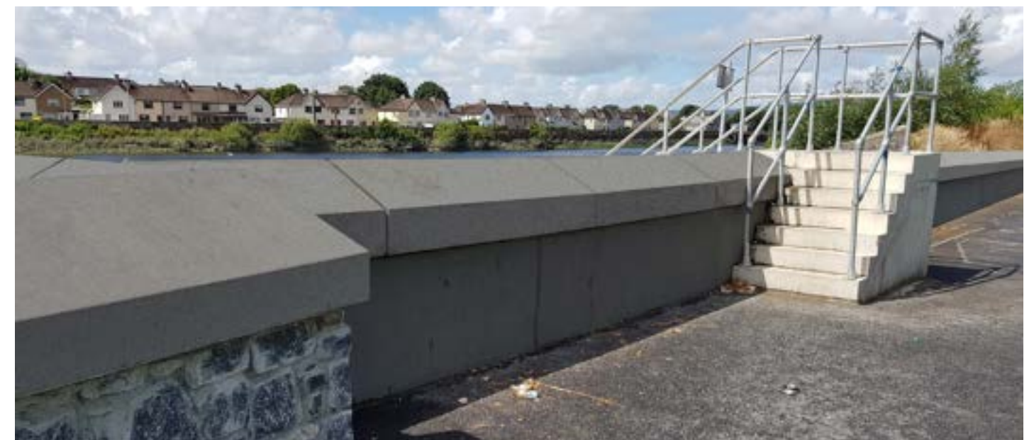
Photomontage showing proposed treatment to existing concrete walling and upgrade of barriers at Verdant Place Steps.
