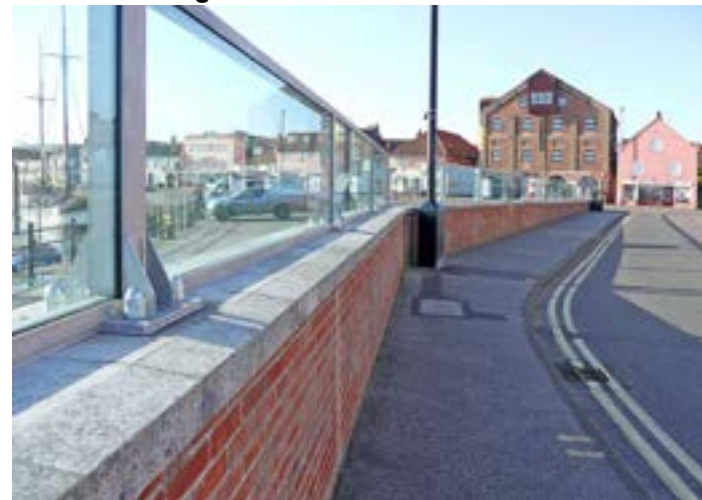
Wels-next-the-sea glass flood wall
