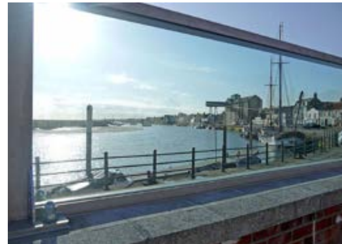
Wels-next-the-sea glass flood wall
