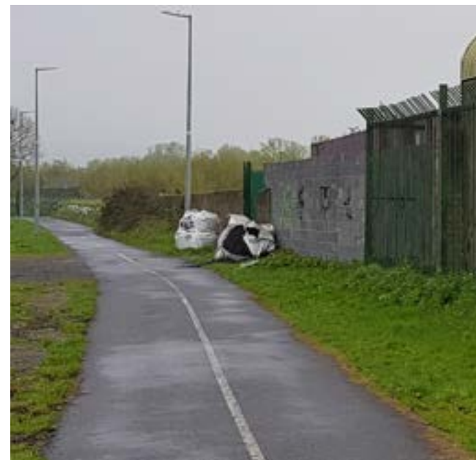
Existing northern section of the Athlunkard boundary.
