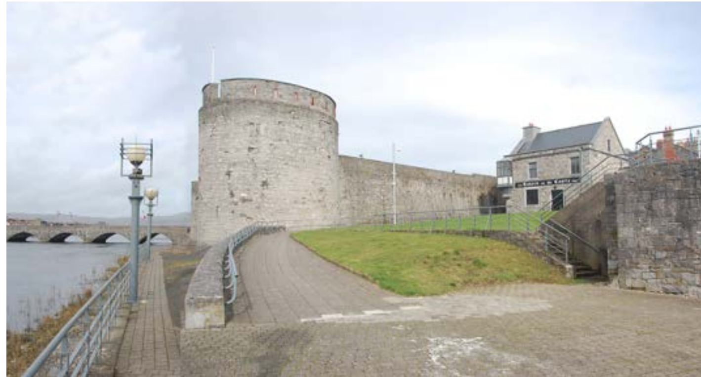
Existing photograph showing the relationship between the Castle and the existing railing.
