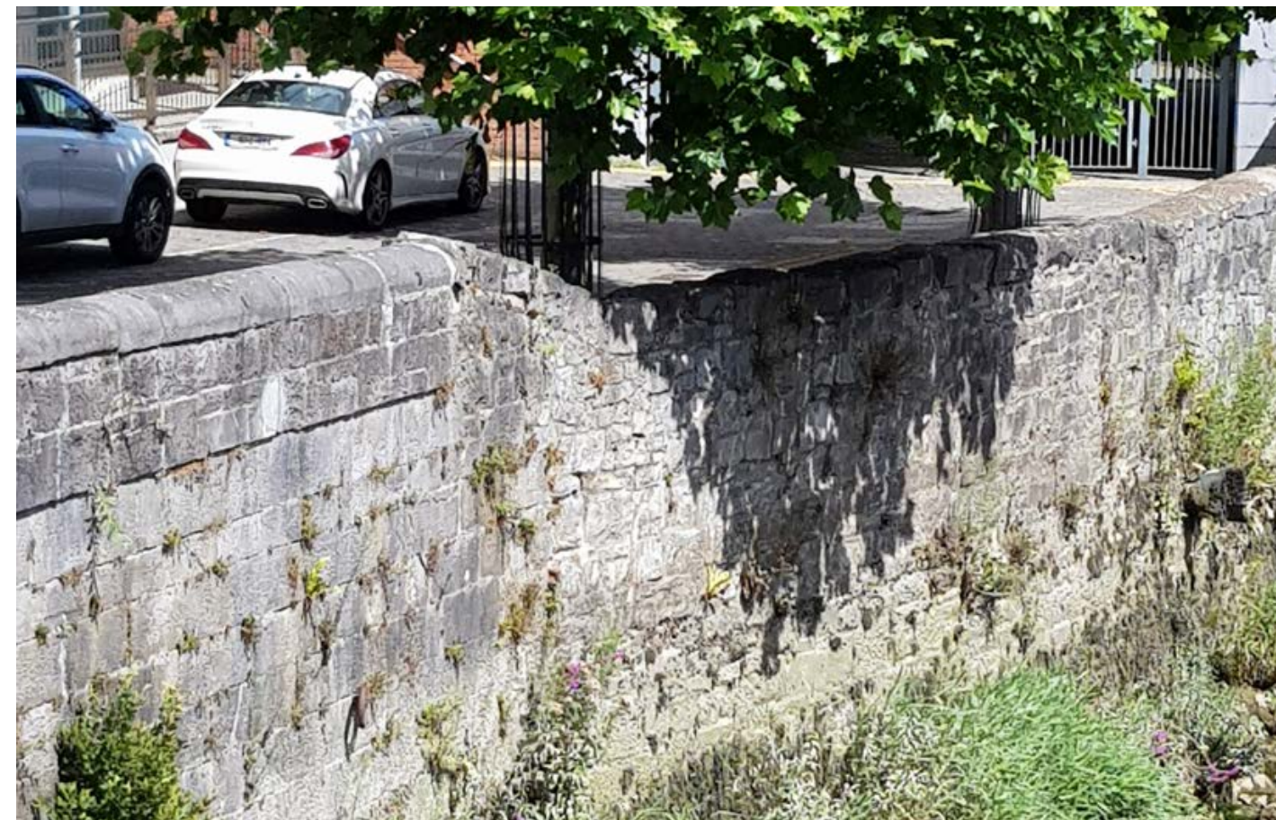
View from Baal's Bridge of the transition in wall styles .
