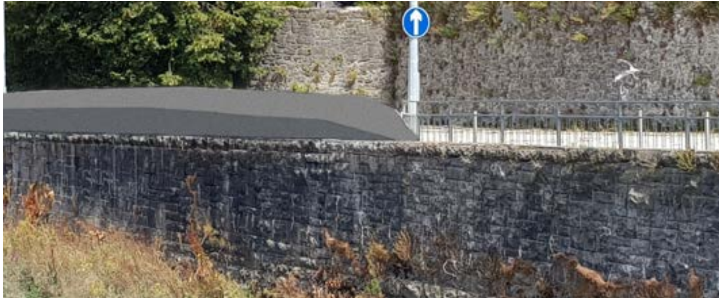
Photomontage showing the exposed concrete sections painted a darker shade of grey.
