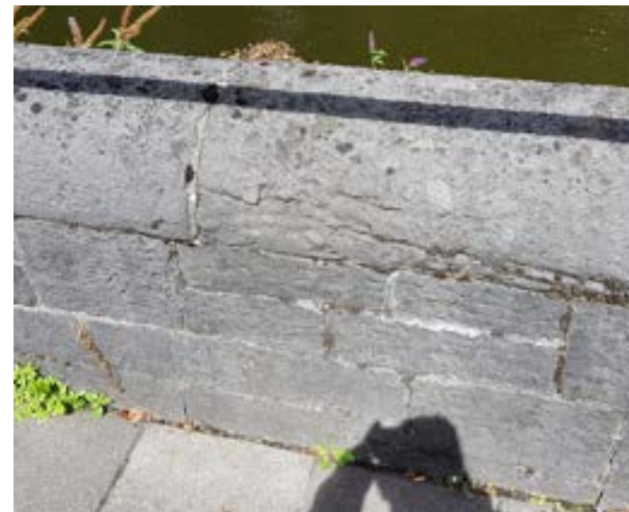
Existing stone wall along eastern section of George's Quay.
