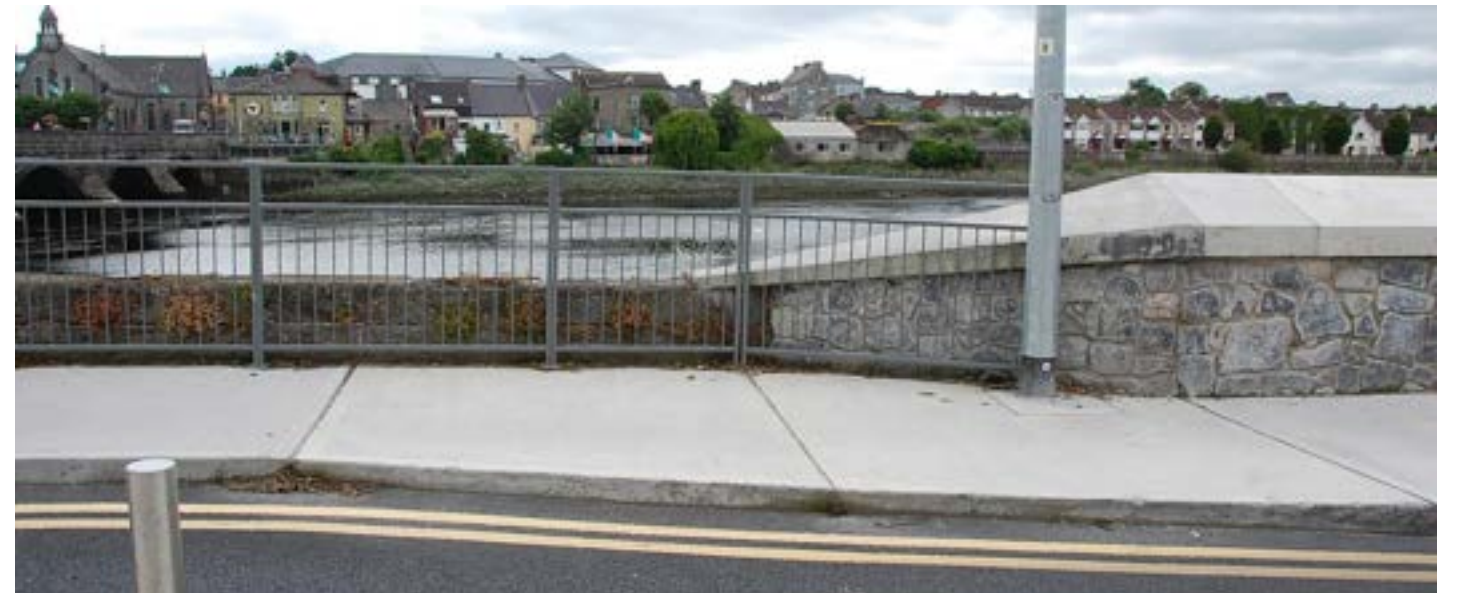
Existing view of the dry-side of the upgraded wall and the existing low wall with safety railing to front.
