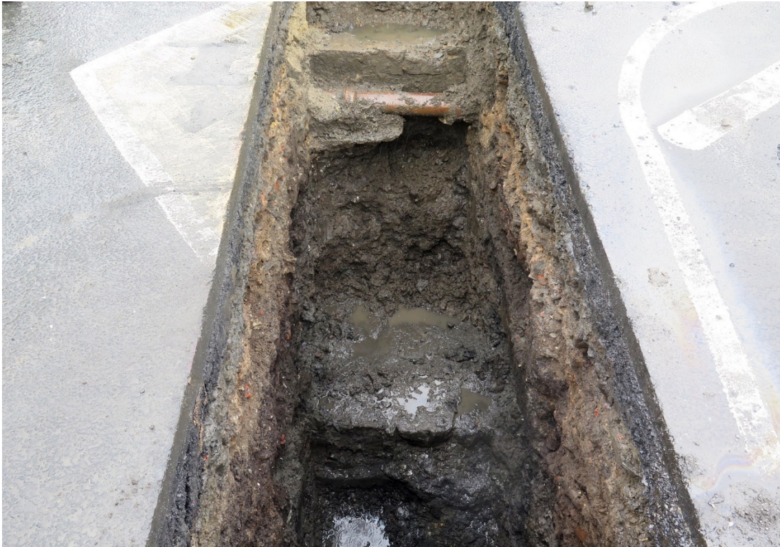
Figure 87 Northeast-facing view of TT5-2C at the completion of excavations
