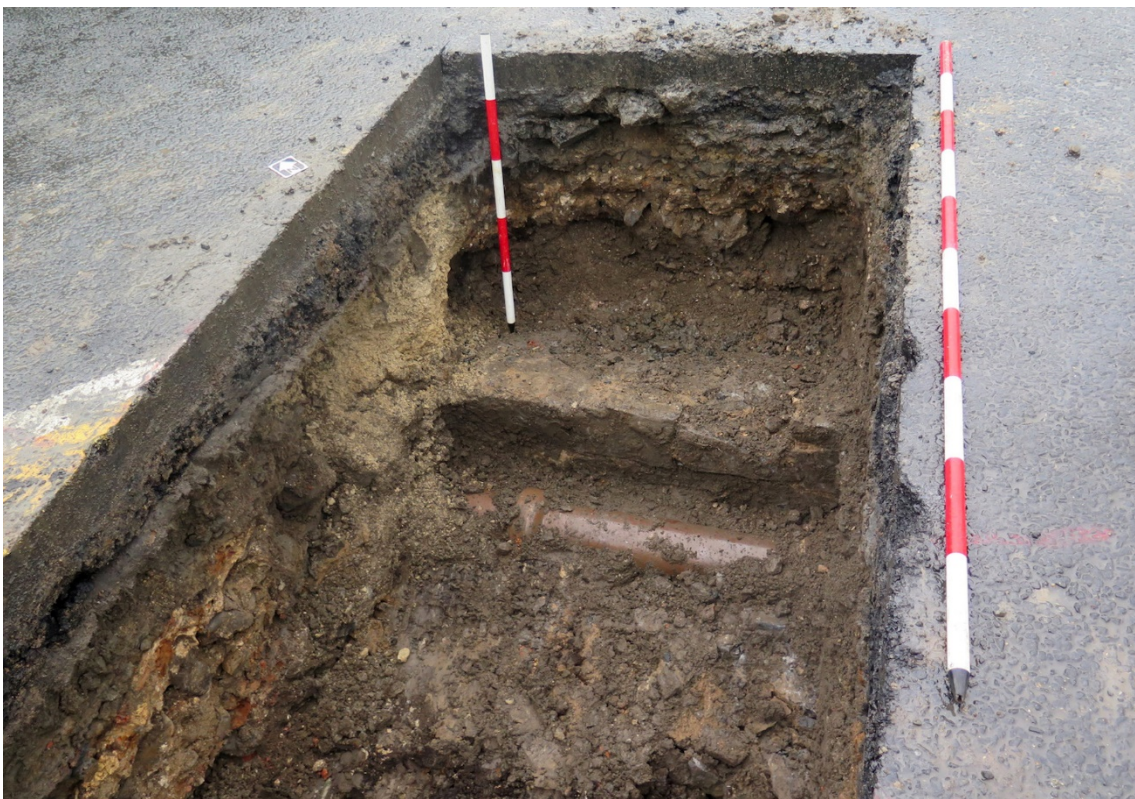
Figure 88 Stone lined culvert for terracotta pipe in the northeast of TT5-2C
