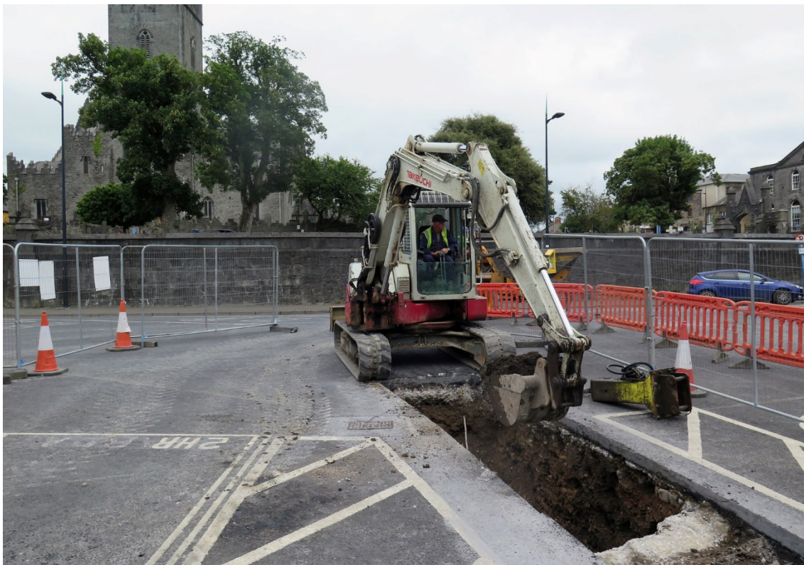
Figure 103 Location of TT5-4, facing northeast towards St Mary's Cathedral
