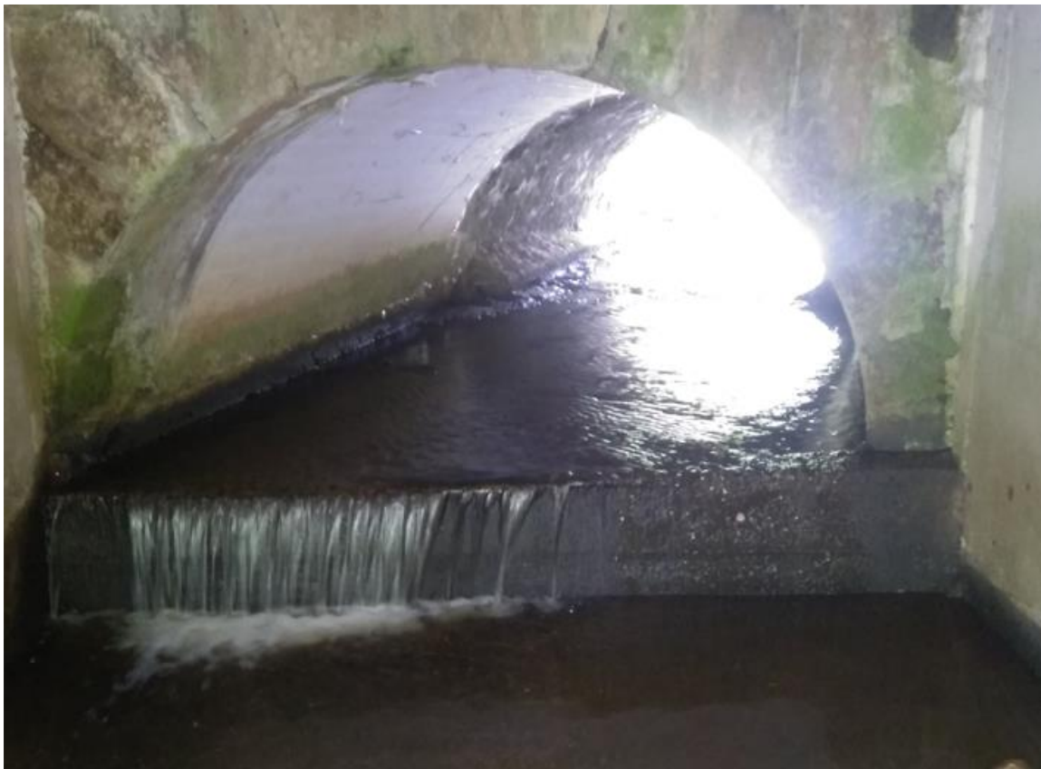
Figure 2.27: Survey Photo of Weir Inside One of the Spring Water Lane Bridge Openings
