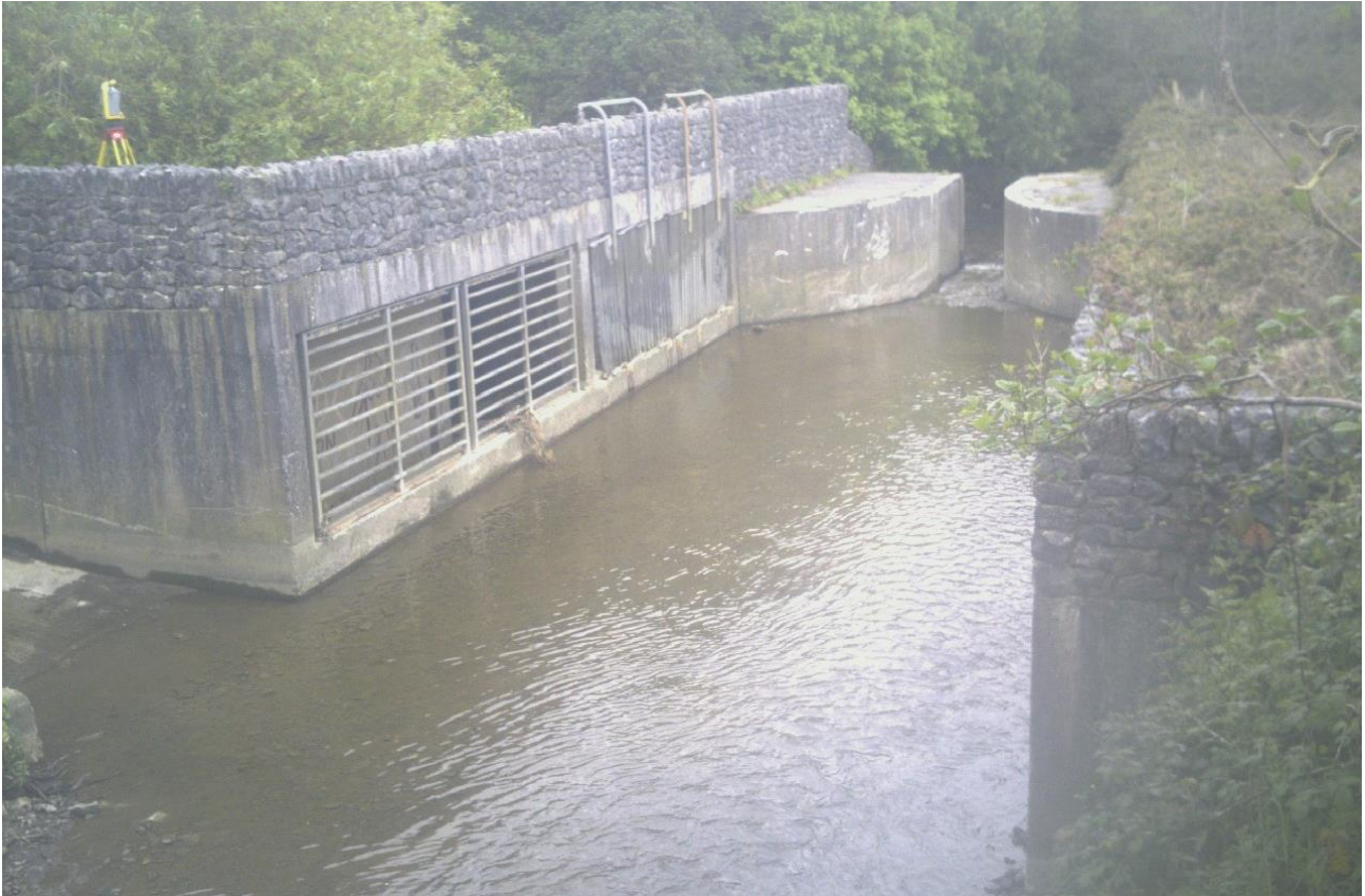
Figure 2.33: Oakpark Road Gauging Station Location Viewed from Upstream, Taken in 2012 Prior to Installation
