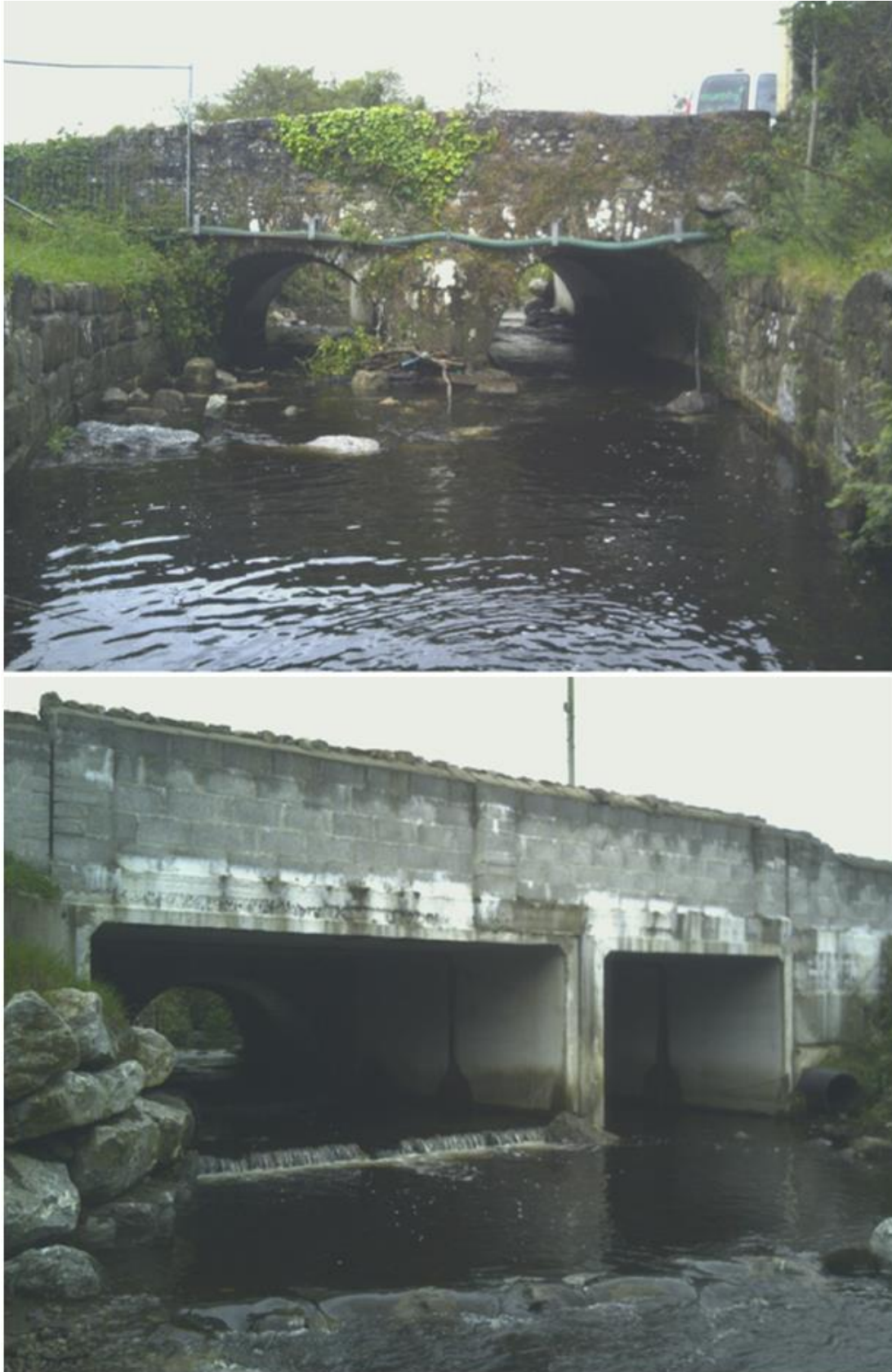
Figure 2.25: Upstream (top) and Downstream (bottom) View of the Spring Water Lane Bridge, taken in 2012 Prior to Installation
