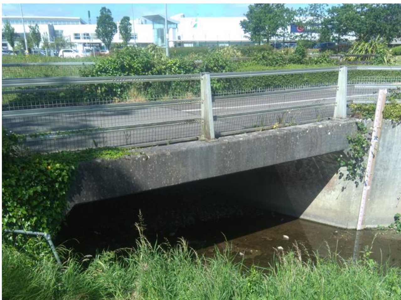
Figure 2.40: Manor West Gauging Station Location Viewed from Upstream
