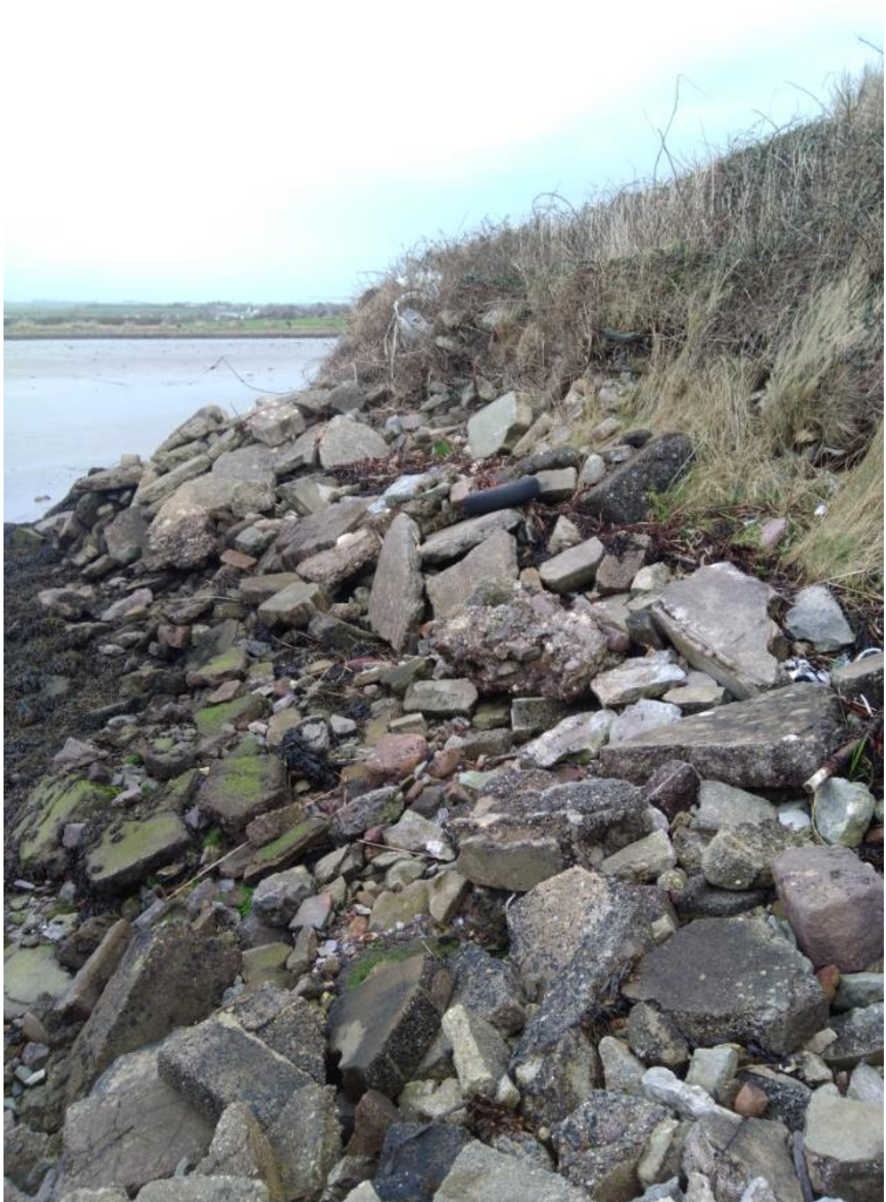
Figure 6.8: Survey Imagery of Blennerville Embankment nearby XS100W
