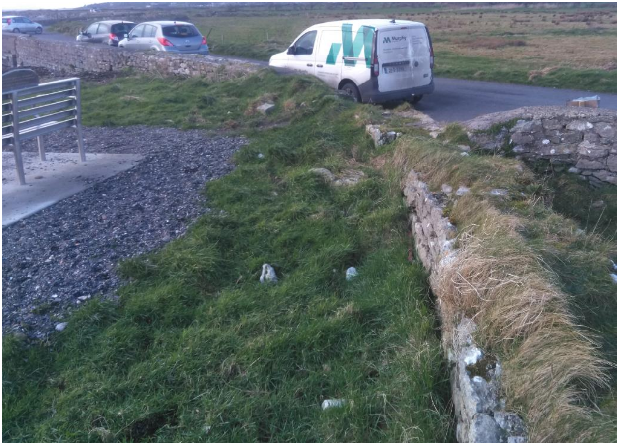
Figure 6.12: Survey Imagery of Wall at North End of Cockleshell Beach Embankment (XS800S)
