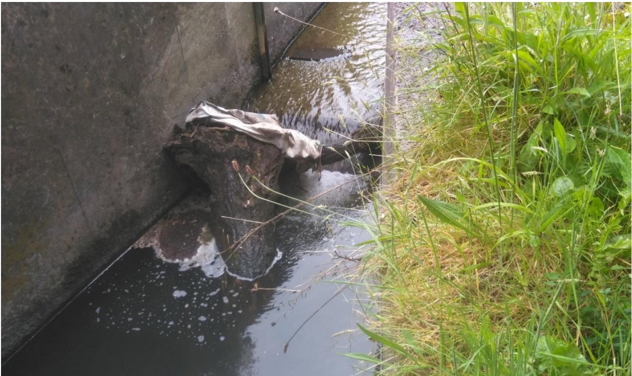
Figure 2.34: Weir Situated 25 m Downstream of the Oakpark Road Gauge
