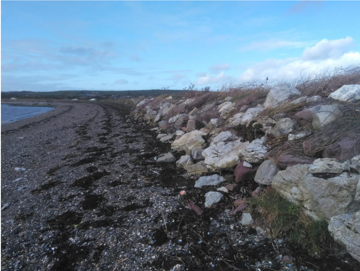
Figure 6.13: Survey Imagery of Cockleshell Beach Embankment in vicinity of XS600
