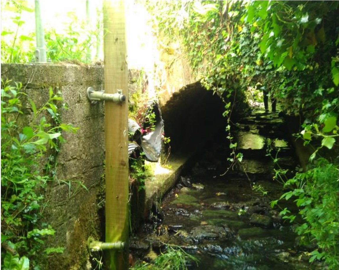
Figure 2.13: Lisloose Gauging Station at Bullock Hill Bridge Viewed from Downstream
