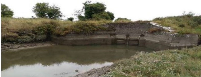
Figure 2 - Flood gates facing southwest.
