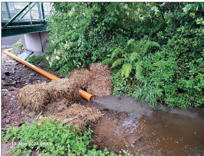
Caption 9 Silt contamination coming from road gullies during rainfall event - Area 2 Cois na Gleann
