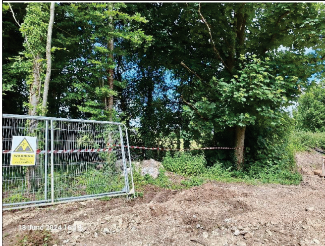
Caption 11 Hazard tape installed around trees to be protected and upheld - Area 3 New Line.
