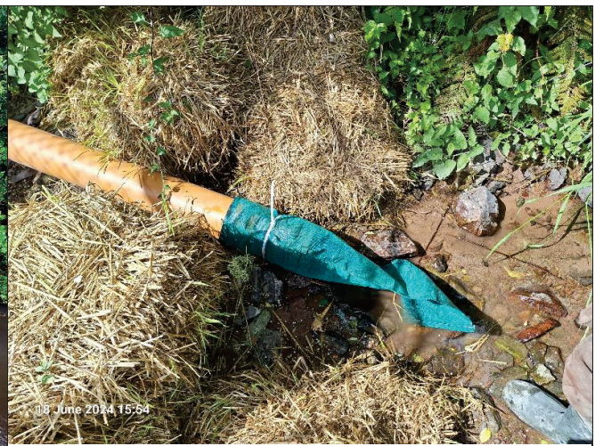
Caption 10 Silt sock installed on outfall pipe of road gullys - Area 2 Cois na Gleann
