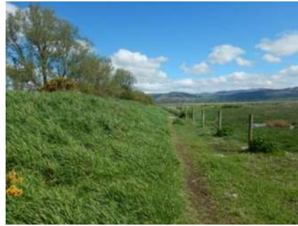
Figure 1 A view of the Lord Limerick embankment and the protected Salt Marshes
