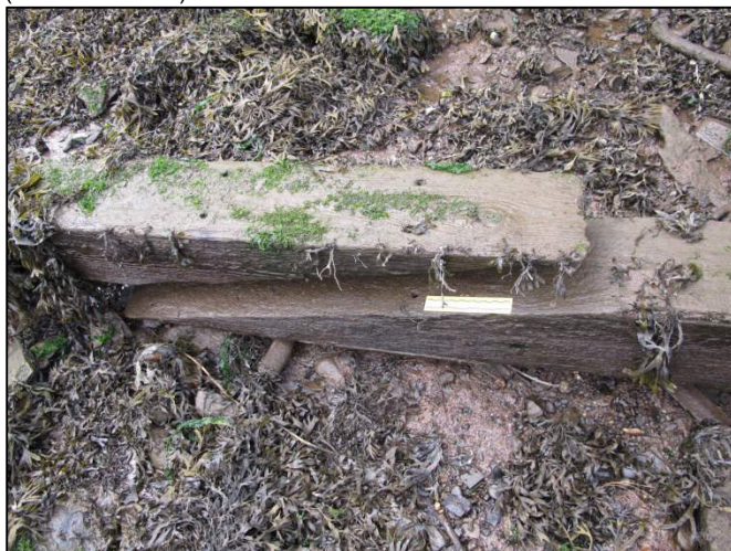
Plate 233: View of scarf-joint between timbers T1-T2 from timber structure (F055) located on intertidal foreshore at Lee Mills (150mm scale).
