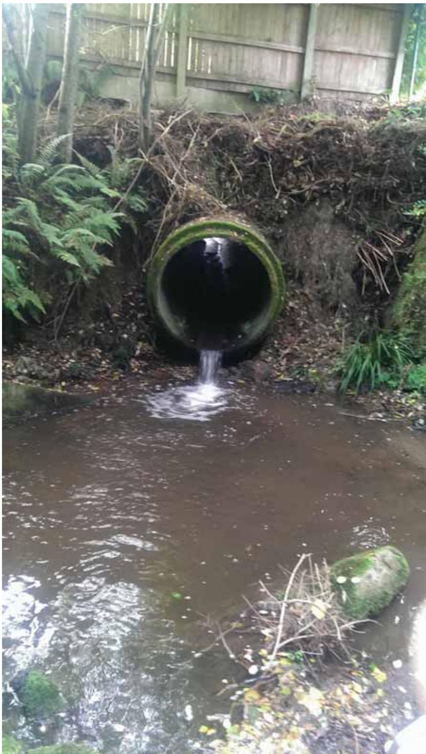
**Photo 2. Plunge pool and pipe which forms a further barrier to fish movement at the upstream end of Site 1.**
