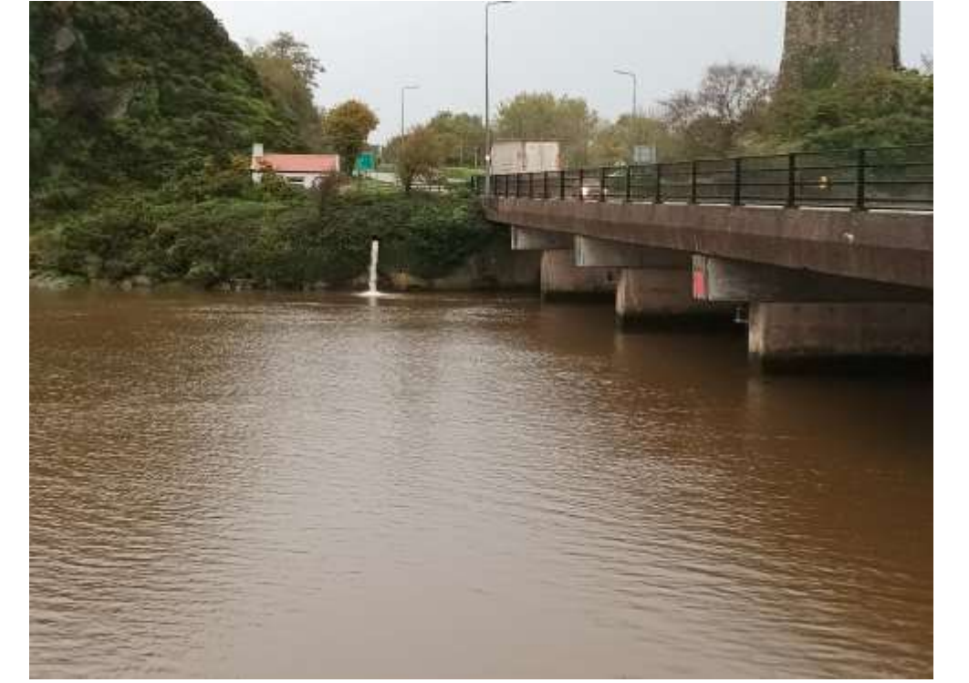
Ferrycarrig bridge area
