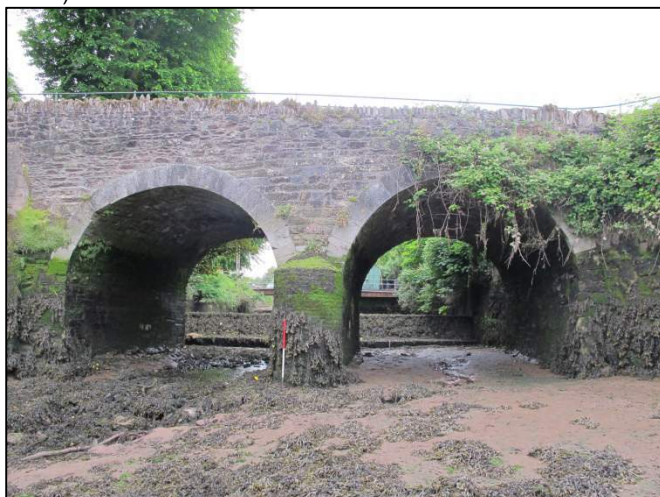
Plate 26: West-facing view of downstream façade of Alderman Reily's Bridge (1m scale).
