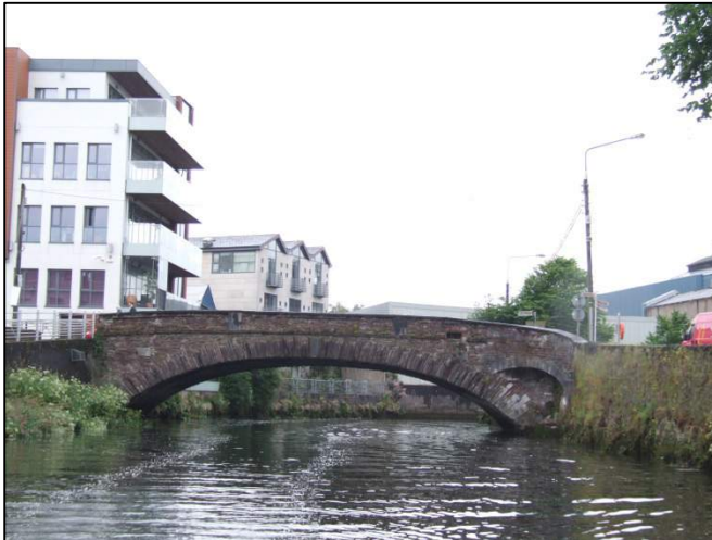
Plate 20: East-facing view of upstream façade of Clarke's Bridge.
