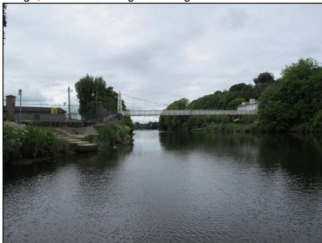
Plate 74: West-facing view of downstream side of Daly Suspension Bridge.
