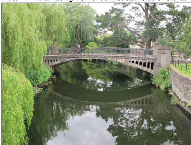
Plate 72: West-facing view of downstream façade of Newman's Bridge.
