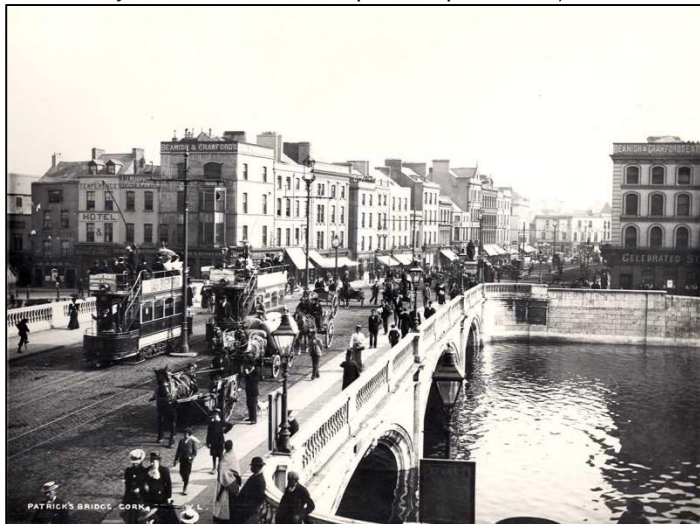
Plate 5: Late nineteenth-century photograph showing trams crossing St. Patricks Bridge (source: www.corkpastandpresnt.ie ).
