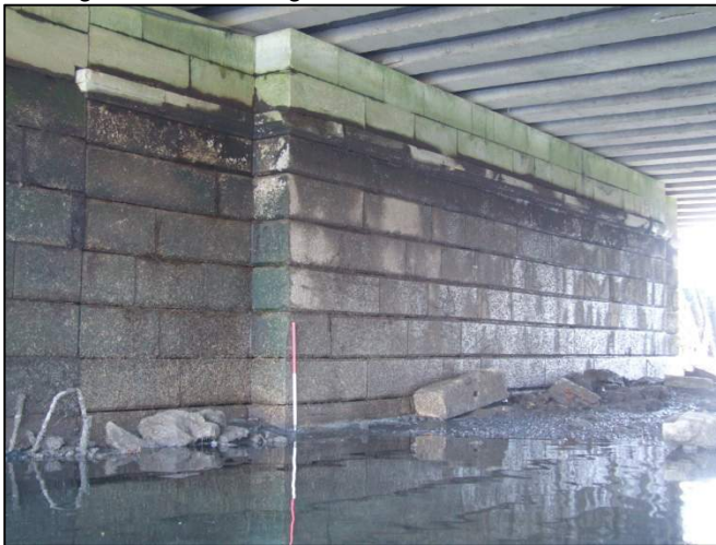
Plate 47: Northeast-facing view showing masonry forming a bridge abutment on the north side of the channel, located beneath the original Parnell Bridge (1m scale).
