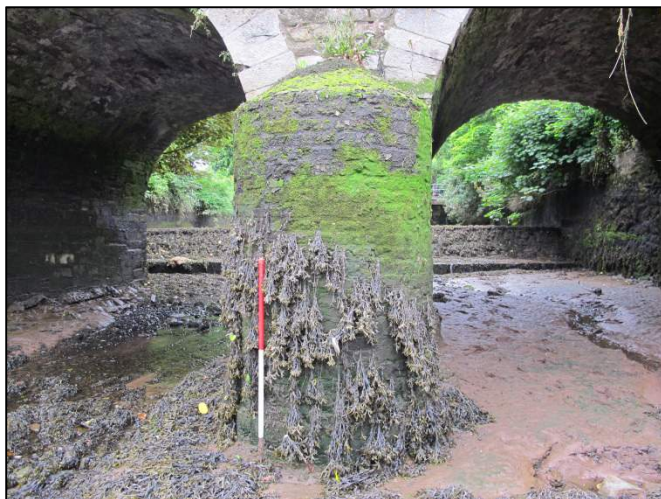
Plate 28: West-facing view of downstream cutwater at Alderman Reily's Bridge (1m scale).
