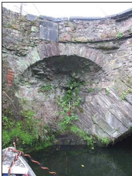
Plate 25: Downstream view of a springing arch added to the south side of the bridge structure in order to widen its approach (1m scale).
