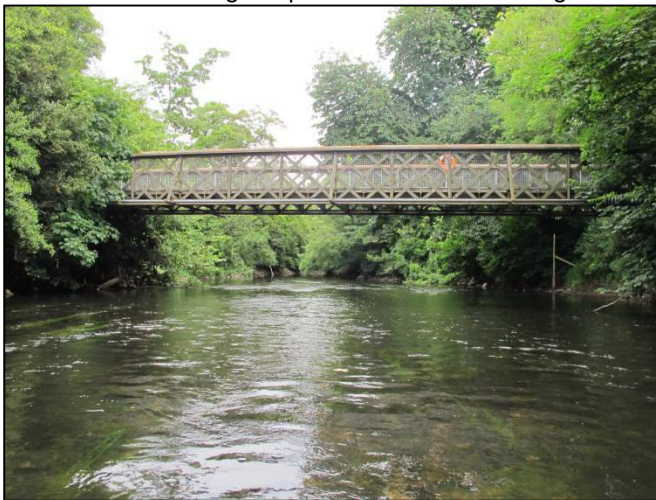
Plate 59: East-facing of upstream side of footbridge F013.
