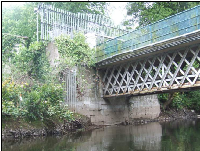
Plate 60: Northeast-facing view of masonry abutment on north side of channel, footbridge F012.
