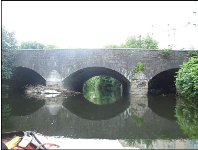
Plate 37: East-facing view of the upstream façade of O'Neill Crowley Bridge (formerly George IV bridge).
