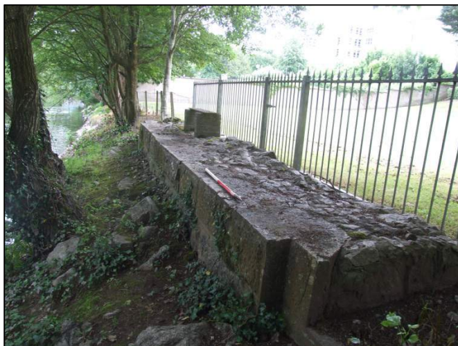
Plate 55: East-facing detail view of remains of masonry bridge abutment located on the south side of channel; bridge site F001 (1m scale).
