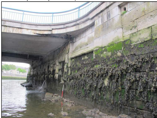
Plate 11: East-facing view of south side of Griffith Bridge showing remnants of previous North Gate Bridge inset into the quay wall (1m scale).
