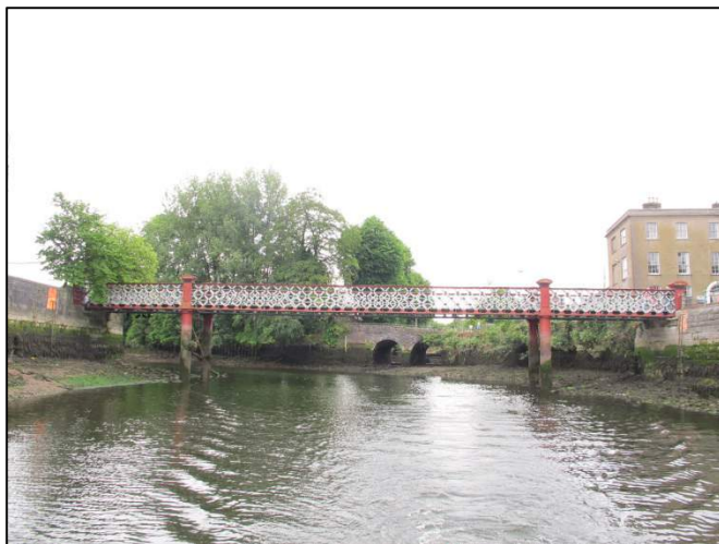
Plate 64: West-facing view of downstream side of St. Vincent's Bridge.
