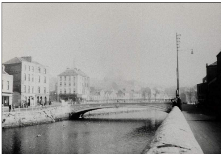
Plate 10: Eighteenth-century photograph showing the upstream side of North Gate Bridge (source: Lawrence Collection www.corkpastandpresent.ie ).
