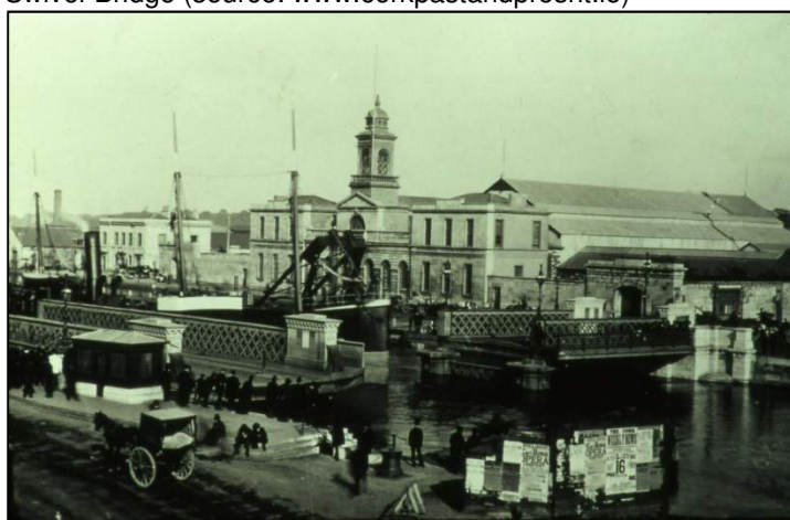
Plate 44: Twentieth-century photograph of the iron swivel-bridge that replaced (1882) the earlier masonry structure forming Anglesea Bridge (source: Cork City Library).
