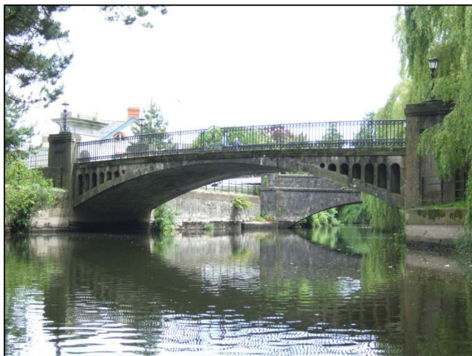
Plate 73: East-facing view of upstream façade of Newman's Bridge, Donavan's Bridge in background downstream.
