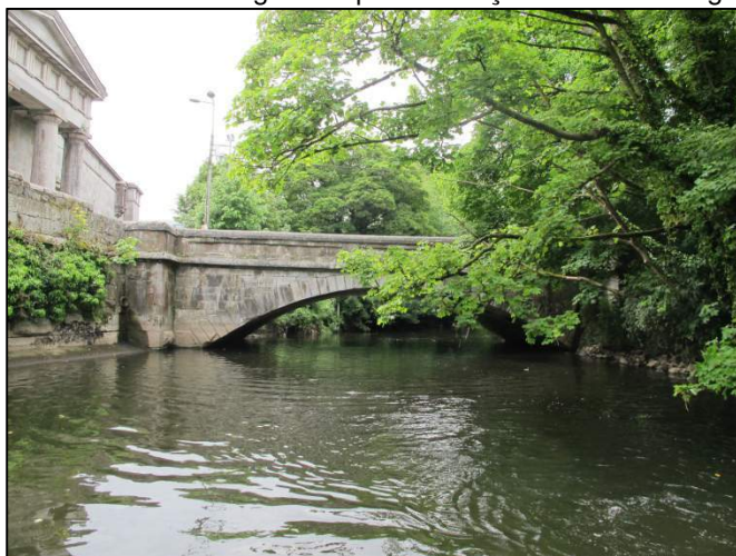
Plate 51: East-facing view downstream façade of Gaol Bridge.
