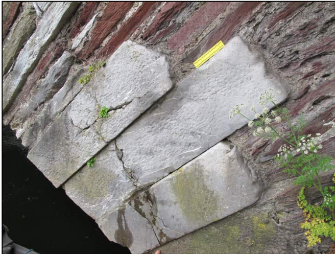
Plate 23: Detail shot of neat-cut limestone used for the arch-ring springing stones at Clarke's Bridge (150mm scale).
