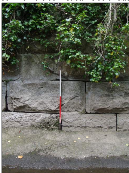
Plate 53: Detail view of masonry used to construct the retaining wall at Gaol Bridge (1m scale).
