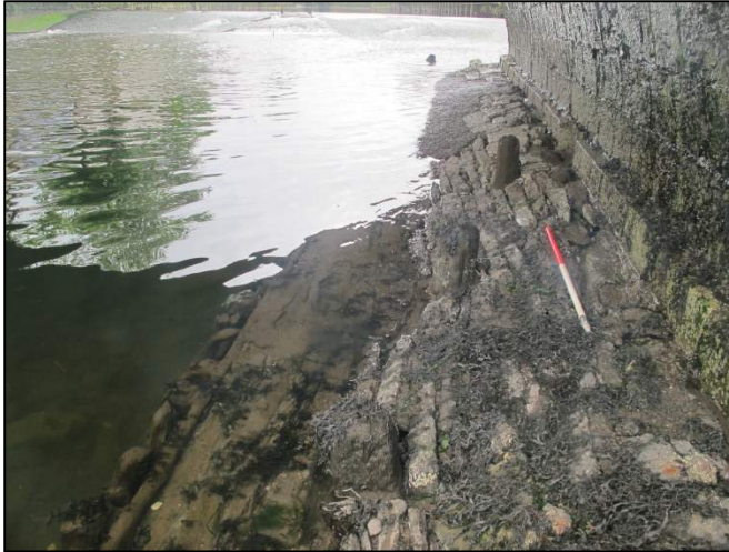
Plate 19: West-facing view timber shuttering and bridge foundations located on north side of archway at Parliament Bridge (1m scale).
