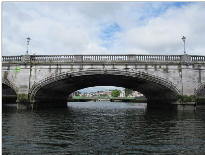
Plate 34: West-facing view of the central (elliptical) archway on downstream side of St. Patrick's Bridge.
