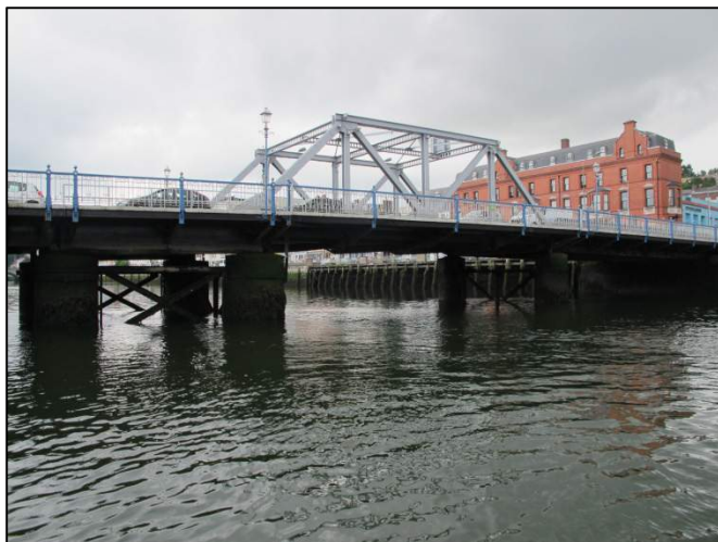
Plate 70: East-facing view of upstream side of Brian Boru Bridge.
