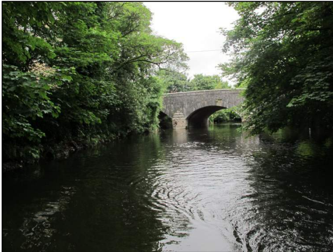
Plate 38: West-facing view of downstream central-arch of O'Neill Crowley Bridge (formerly George IV bridge).
