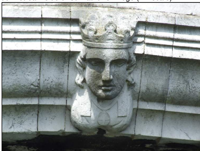
Plate 36: Detail view of effigy on key-stone from southern arch on the upstream side of St. Patrick's Bridge.
