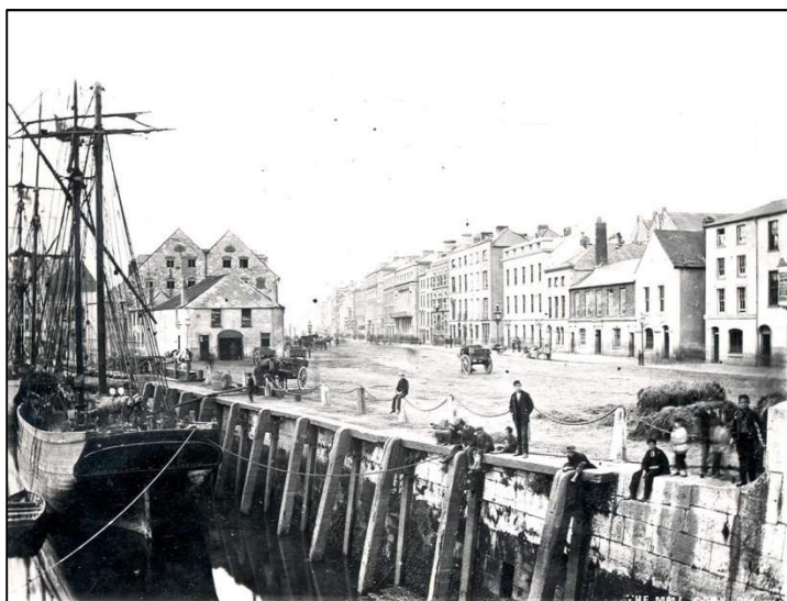
Plate 1: Nineteenth-century photograph showing downstream side of Morrison's Quay and the newly reclaimed South Mall area (source: Lawrence Collection , www.corkpastandpresent.ie ).
