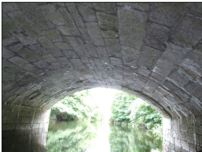
Plate 40: View of the intrados of the central-arch of O'Neill Crowley Bridge (formerly George IV bridge).
