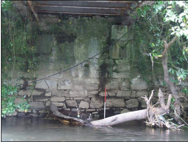
Plate 61: South-facing view of masonry abutment on south side of channel, footbridge F013 (1m scale).
