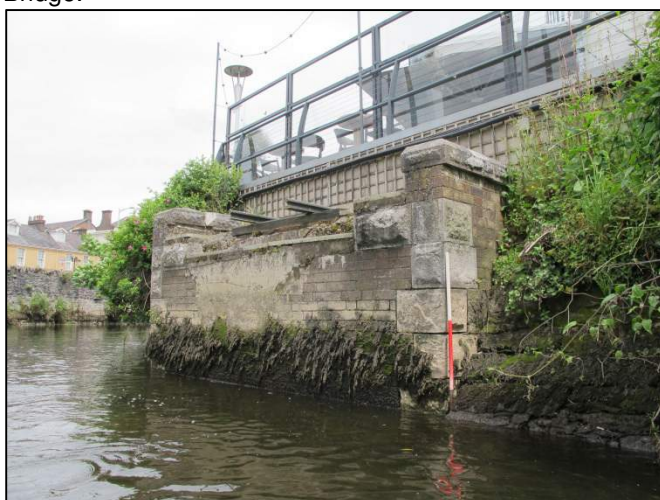
Plate 66: North-facing view of railway bridge abutment at bridge site F16 (1m scale). Note, narrow gauge railway track still protruding from structure.
