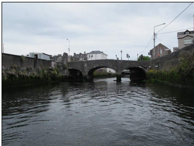
Plate 13: East-facing view of upstream façade of South Gate Bridge.
