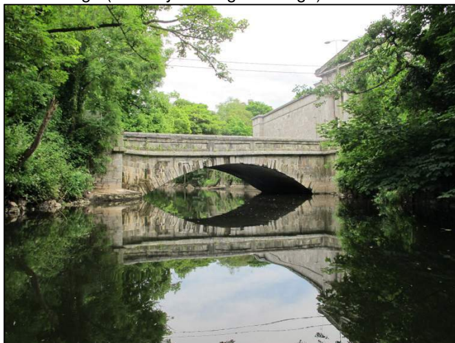
Plate 50: East-facing view upstream façade of Gaol Bridge.
