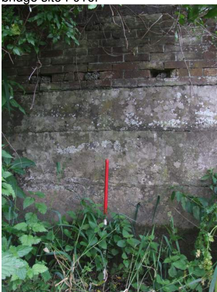
Plate 68: West-facing view bridge abutments of west side of the channel at site F016 (1m scale).
