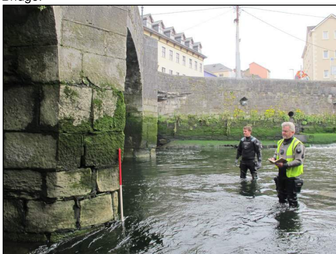
Plate 15: South-facing view of upstream cutwater on South Gate Bridge.
