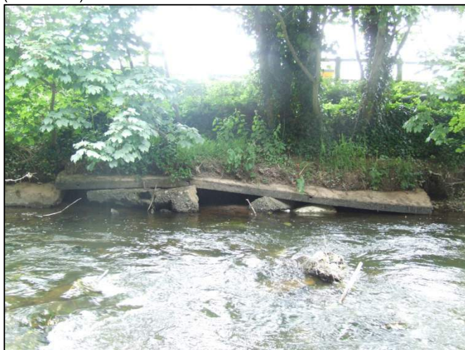
Plate 56: North-facing view of concrete and rocks armour forming north side of the channel at the bridge location.
