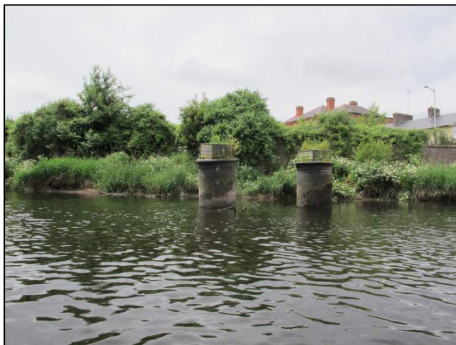
Plate 67: West-facing view of tubular steel bridge supports at bridge site F016.
