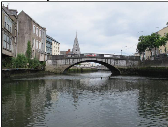
Plate 17: East-facing view of upstream façade of Parliament Bridge.
