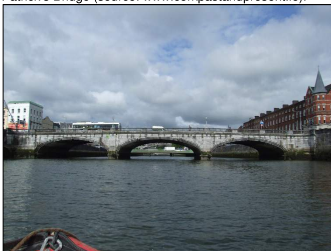
Plate 33: West-facing view of the downstream façade of St. Patrick's Bridge.
