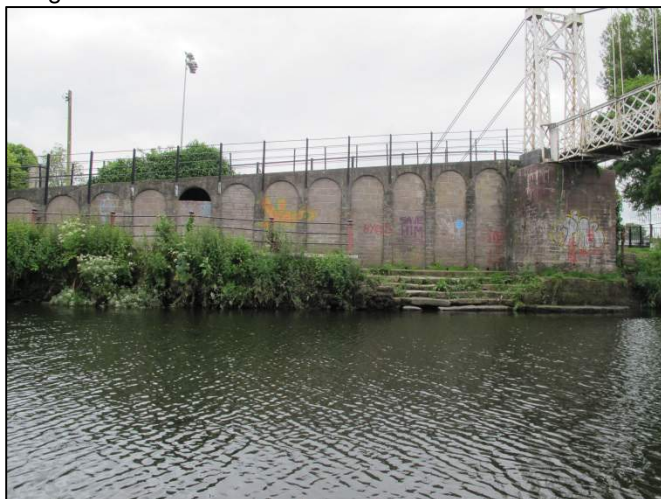
Plate 75: South-facing view of southern bridge abutment and arched access ramp to Daly Suspension Bridge.
