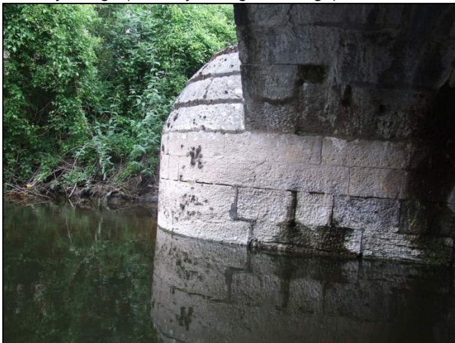
Plate 39: South-facing view of downstream cutwater on O'Neill Crowley Bridge (formerly George IV bridge).
