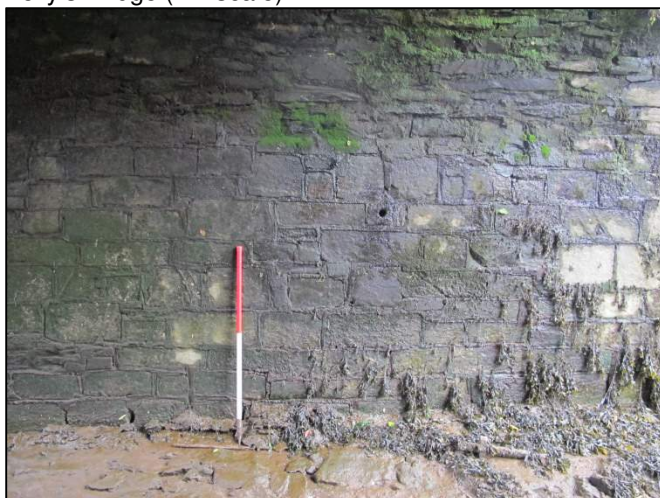
Plate 27: View of arch-wall on the south side of the northern archway at Alderman Reily's Bridge (1m scale).
