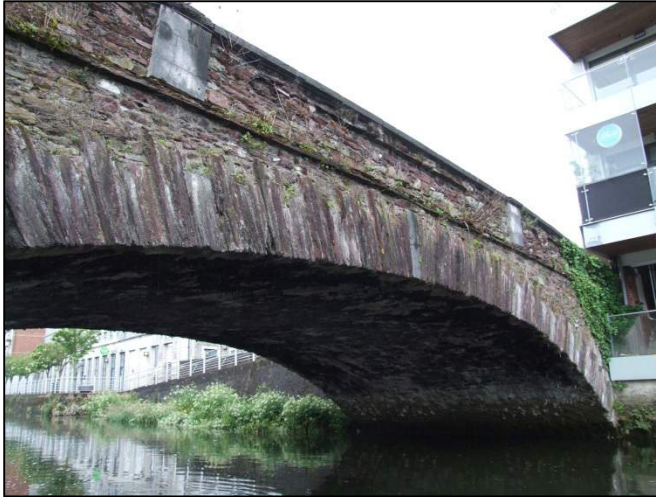
Plate 22: North-facing view of across the arch-ring on the downstream side of Clarke's Bridge.
