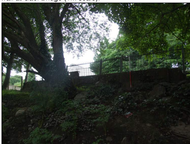
Plate 54: South-facing view of remains of masonry bridge abutment located on the south side of channel; bridge site F0011 (1m scale).
