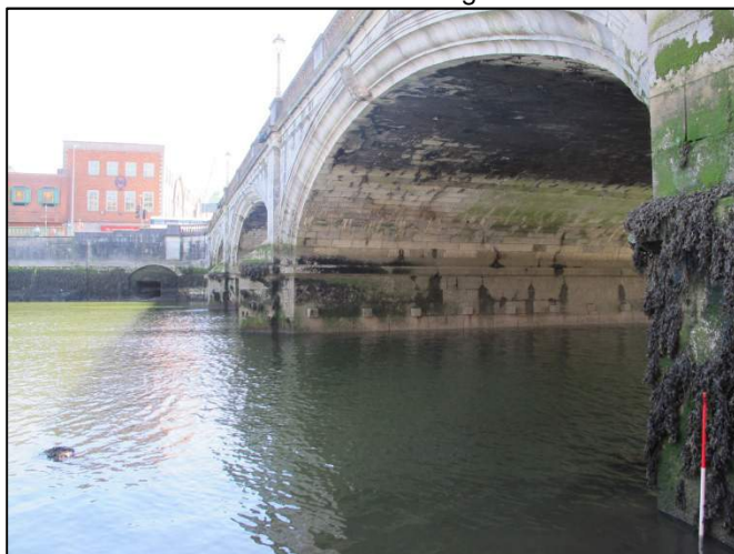
Plate 35: South-facing view of the elliptical archways on the downstream side of St. Patrick's Bridge (1m scale).
