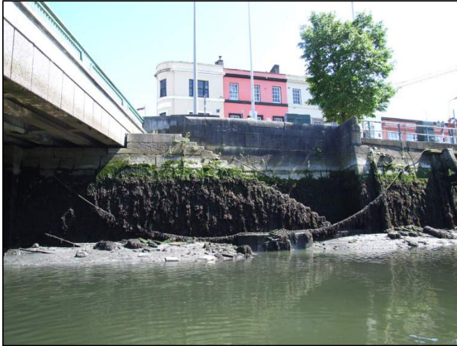
Plate 46: South-facing view showing masonry steps built as part of the original Parnell Bridge.
