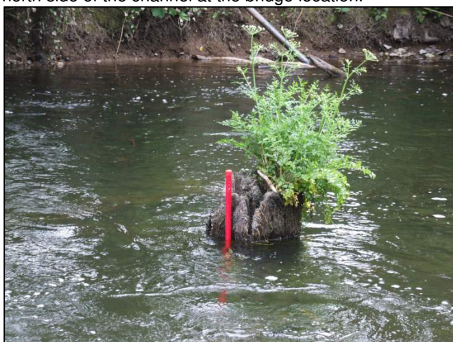
Plate 57: Example of one of the three, square-section, in-river timber piles at bridge site F001.
