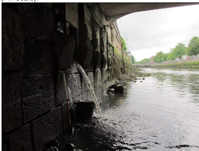
Plate 12: West-facing view of remnants of previous North Gate Bridge inset into the quay wall beneath Griffith Bridge (1m scale).
