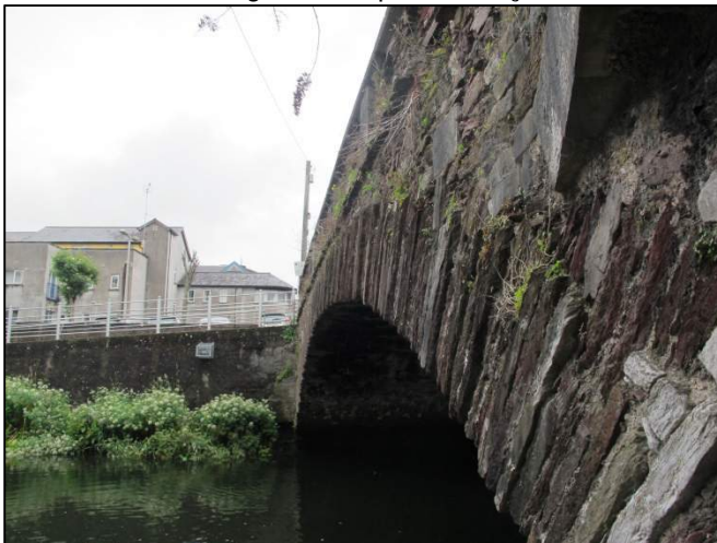
Plate 21: South-facing view across the bridge façade of the downstream side of Clarke's Bridge.
