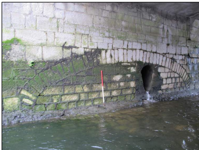
Plate 16: Northeast-facing view of arched-culvert located beneath South Gate Bridge (1m scale).
