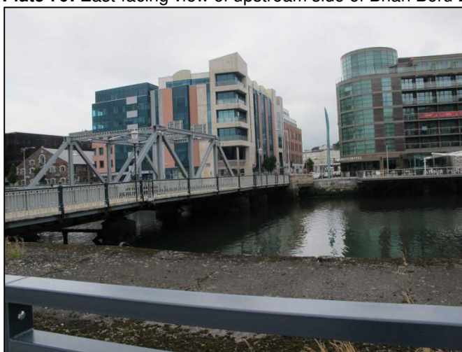
Plate 71: North-facing view of downstream side of Clontarf Bridge.
