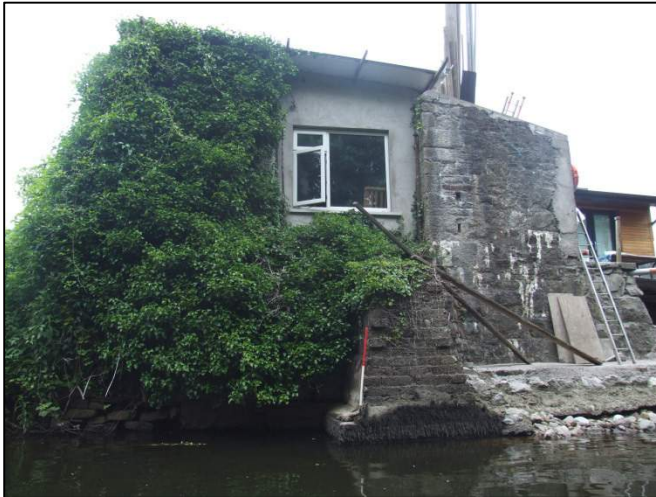
Plate 62: North-facing view of masonry abutment on north side of channel at bridge location F014 (1m scale).
