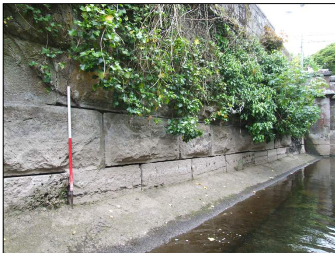
Plate 52: Southwest-facing view across retaining wall that extends 36m from the downstream side of Gaol Bridge (1m scale).
