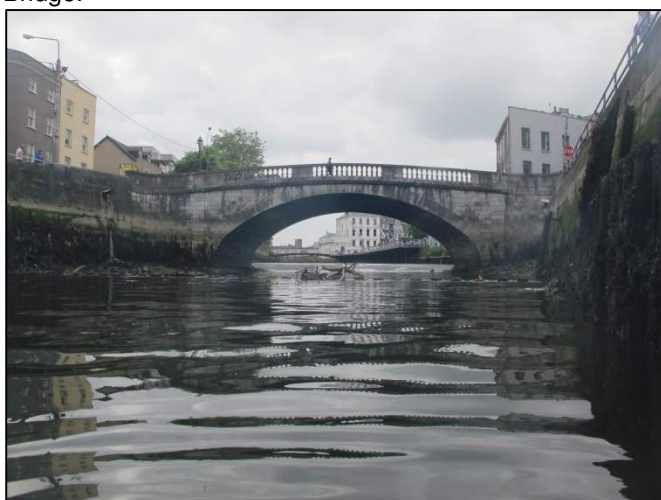
Plate 18: West-facing view of downstream façade of Parliament Bridge.
