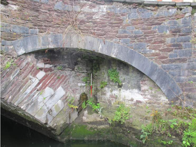
Plate 24: Upstream view of a springing arch added to the south side of the bridge structure in order to widen its approach (1m scale).
