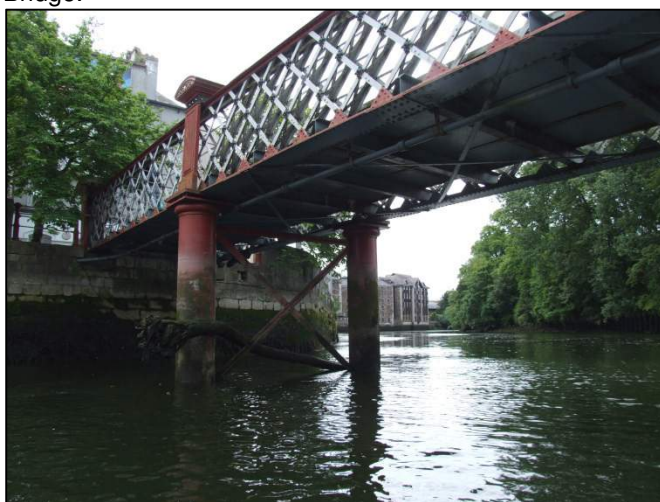
Plate 65: South-facing view showing the underside of St. Vincent's Bridge.
