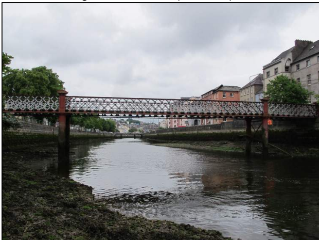
Plate 63: East-facing view of upstream side of St. Vincent's Bridge.
