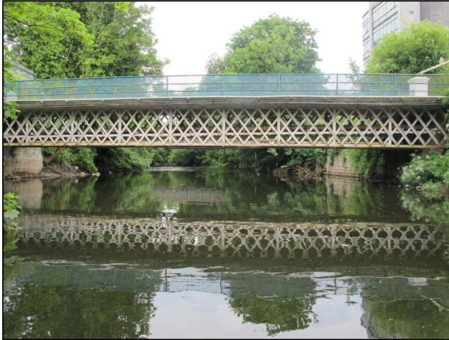
Plate 58: East-facing of upstream side of footbridge F012.
