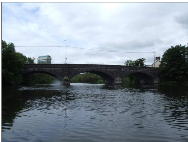
Plate 49: West-facing view of the downstream façade of Thomas Davis Bridge (formerly Wellington Bridge).
