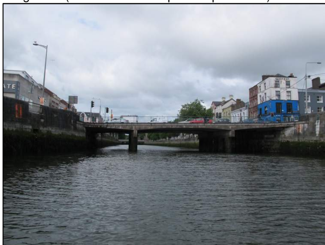
Plate 9: West-facing view of the downstream side of Griffith Bridge.
