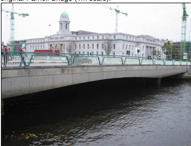
Plate 48: North-facing view upstream side of the modern Parnell Bridge built in 1971.
