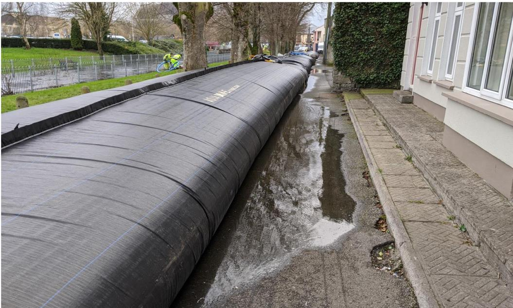
**Figure 31: Temporary flood barrier at Sli na hAbhann**
