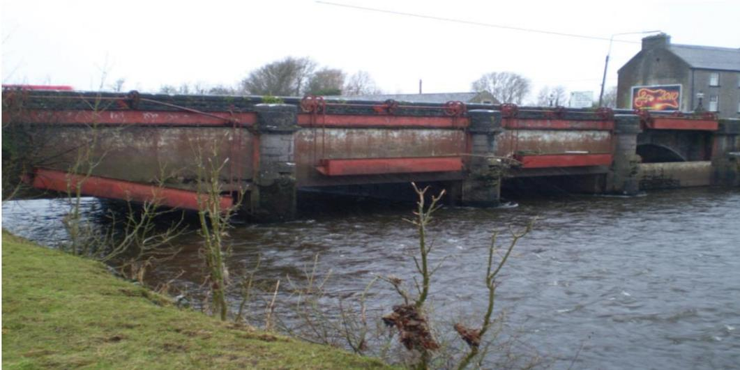
**Figure 24: Sluice Gates on the upstream face (non - flood conditions)**
