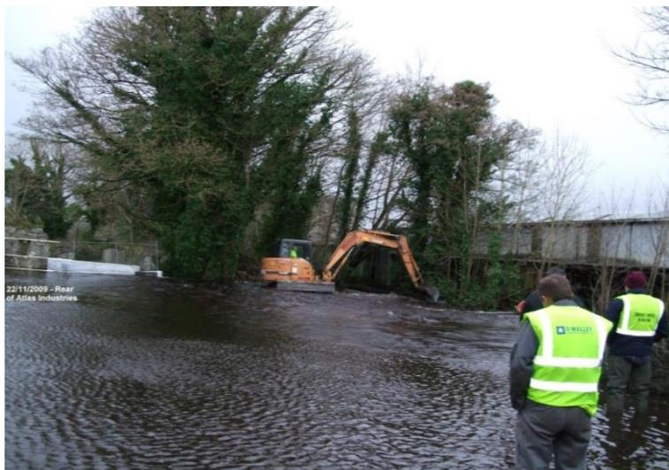
**Figure 45: Removal of the obstruction at the Atlas channels**
