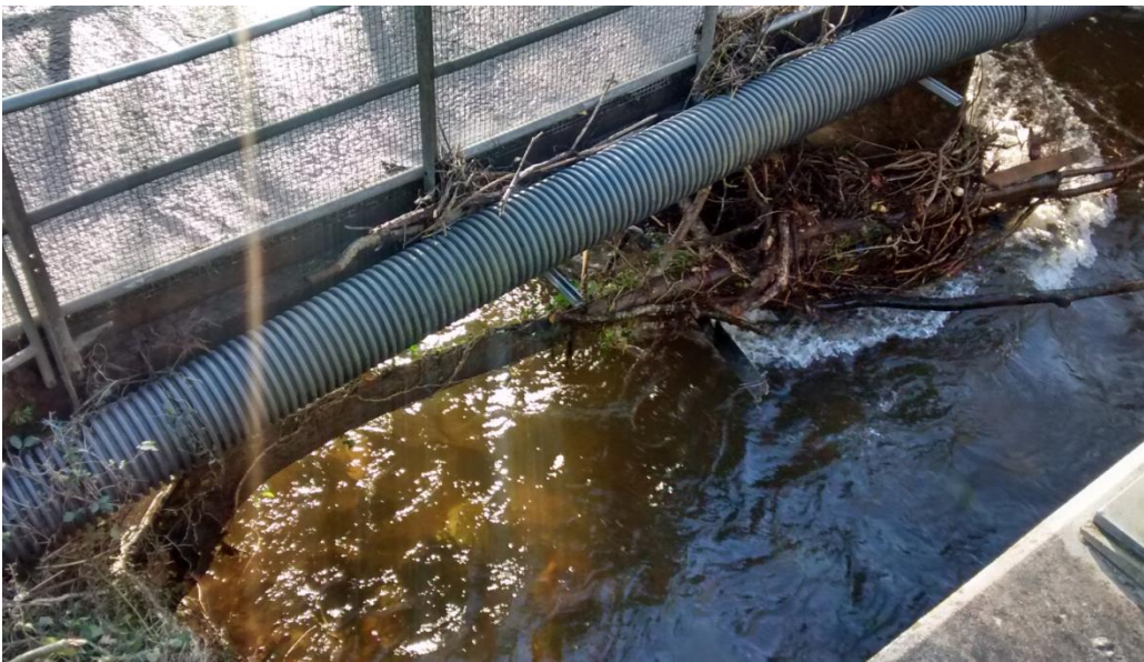
Figure 5.11 Blockage at Moore's Bridge
