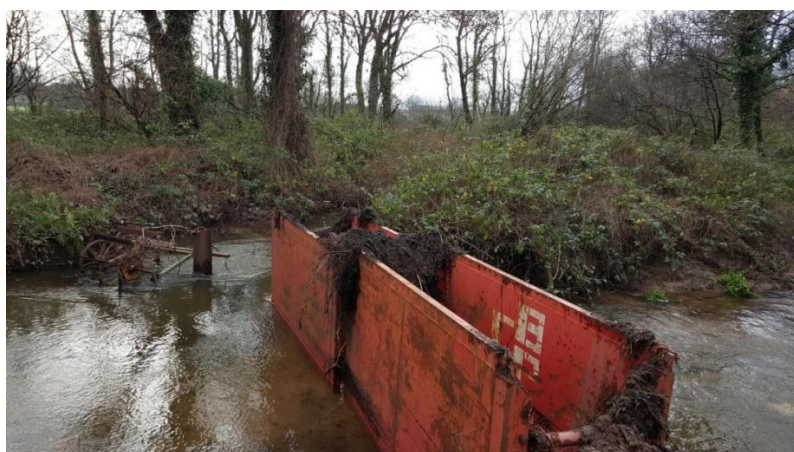
Figure 5.24 Photo of trench box installed by CCC to limit the inflow to the millrace
