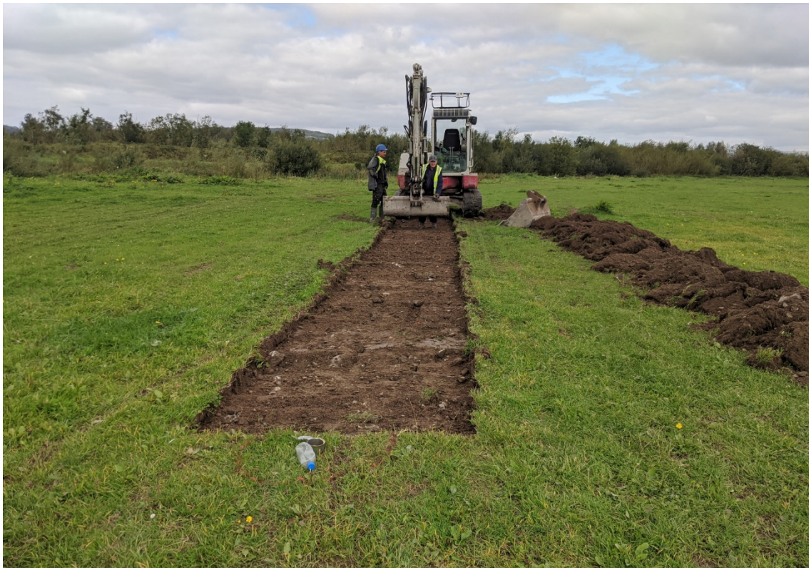
Figure 181 East-facing view along TT9-3.
