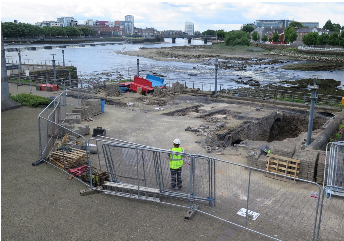
Figure 16 Excavations in Area 1, facing southwest down the River Shannon
