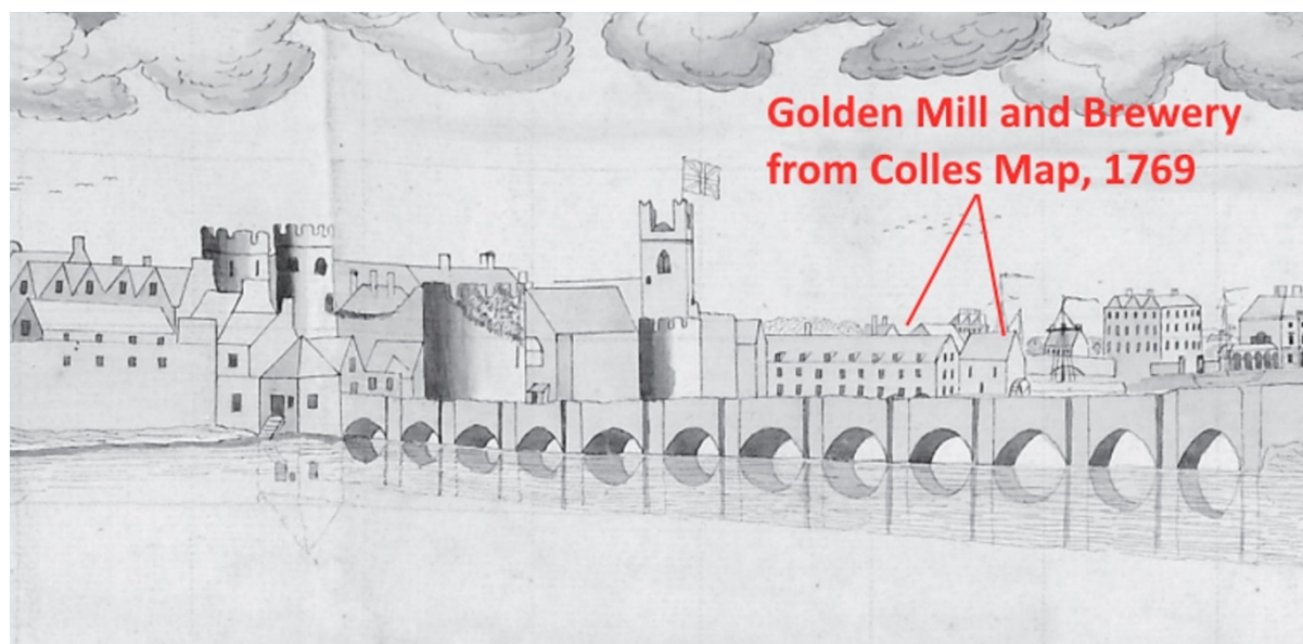
Figure 6 Illustration from Colles's Map of Limerick 1769 showing mill with wheel and brewery.
