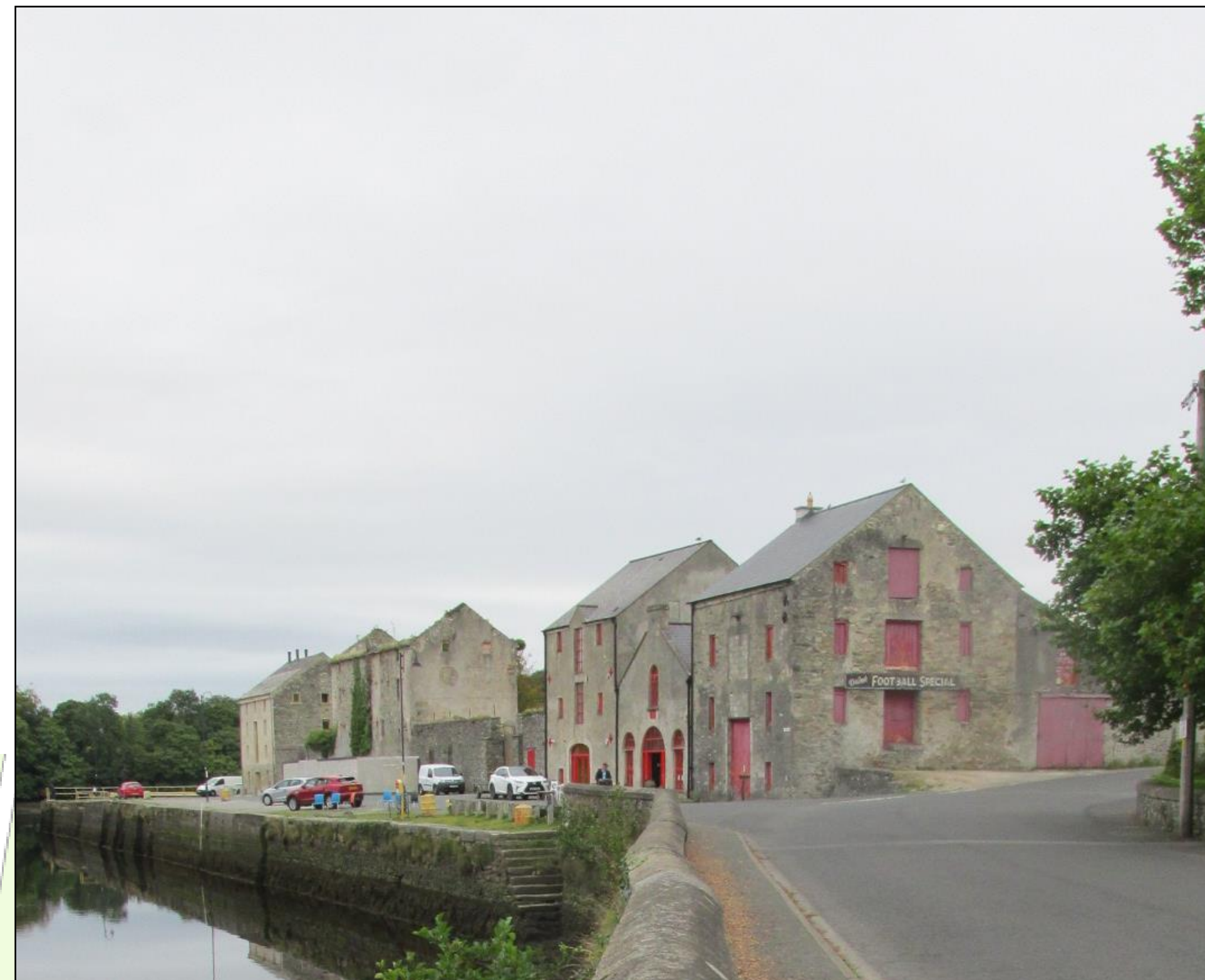
Protected buildings on the Quays as seen from Shore Road
