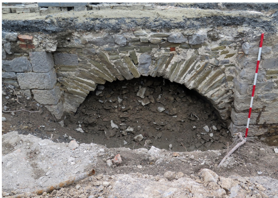
Figure 26 Arch of barrel vaulted tunnel in TT1-1 (C1-1-06)
