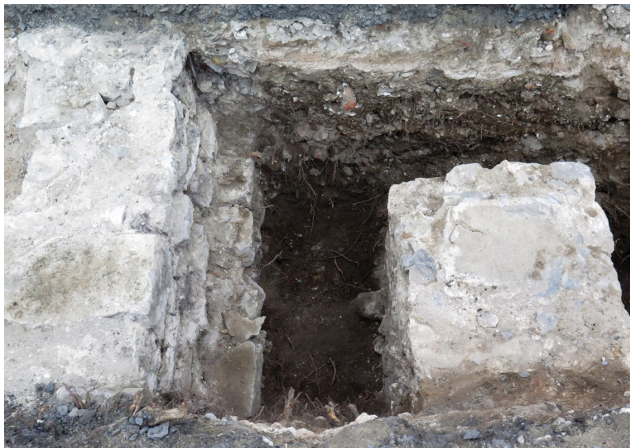
Figure 30 Abutment wall of barrel vault in TT1-3 (C1-3-14)
