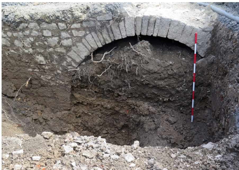
Figure 25 Arch of barrel vaulted tunnel in TT1-1 (C1-1-05)
