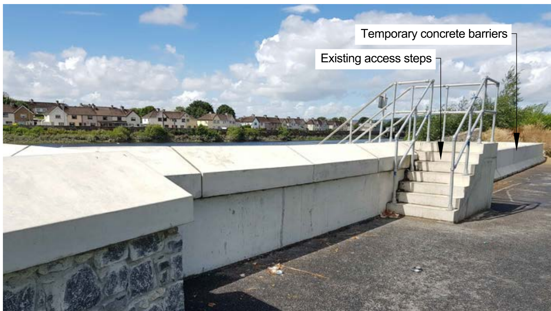
Existing concrete walling and barriers at Verdant Place Steps (KIFRS-A-001)
