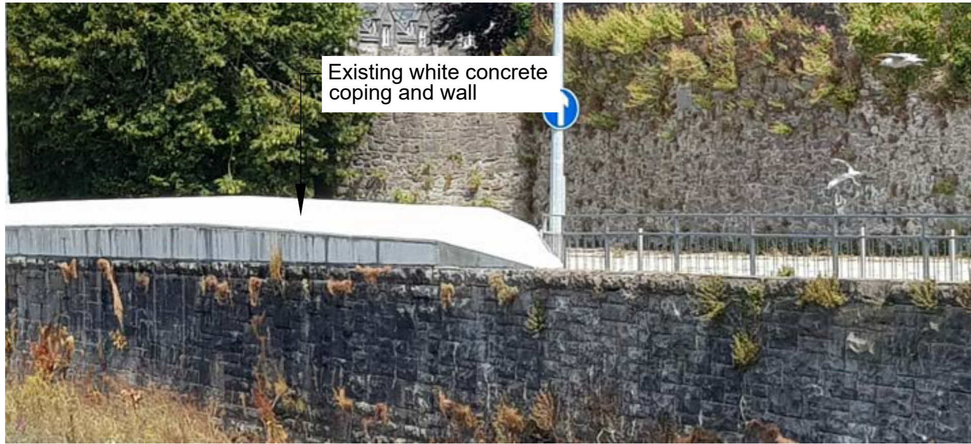
Existing concrete coping and walling along Verdant Place (KIFRS-A-001)
