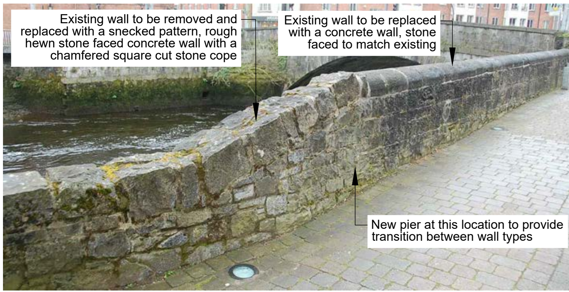
Wall treatment along the southern end of Sir Harry's Mall (KIFRS-A-009)
