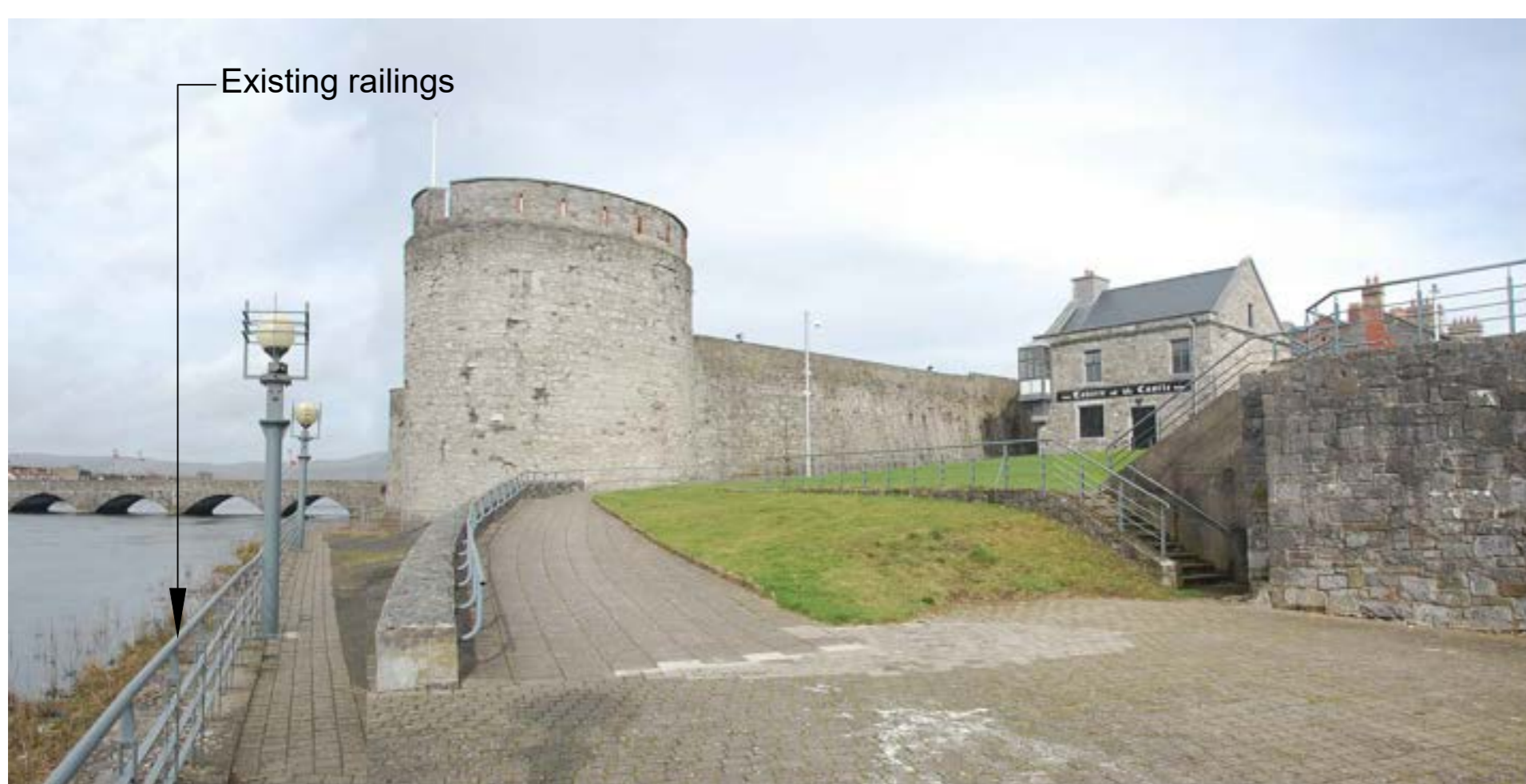
Existing quay edge railing south of King John's Castle (KIFRS-A-010)
