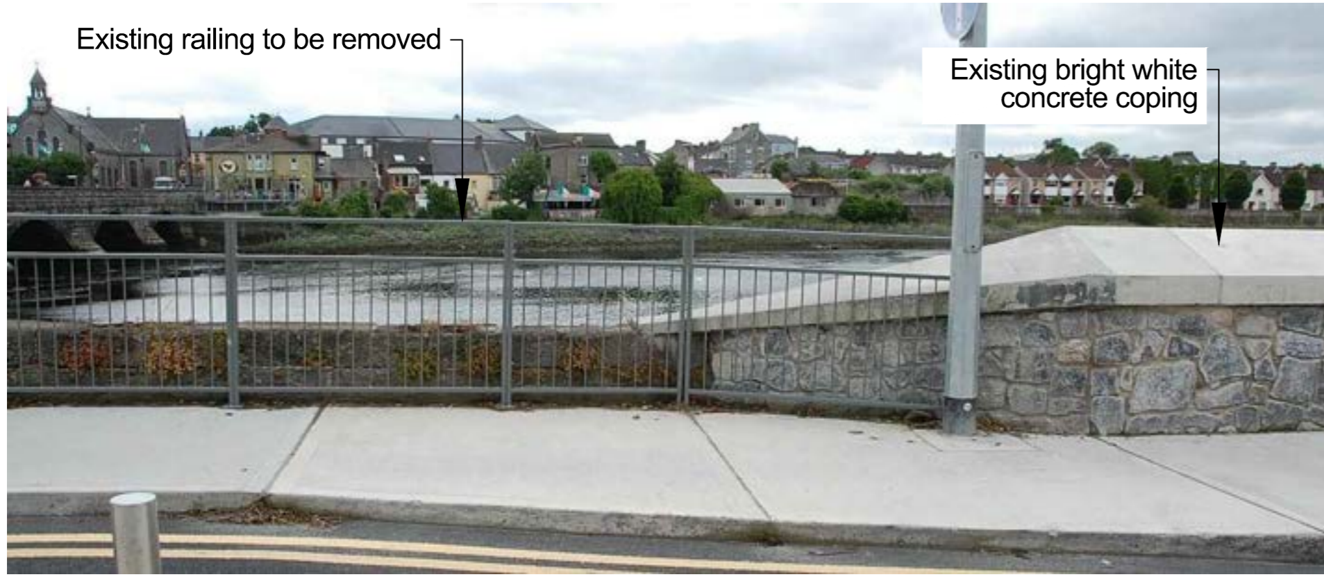
Existing railing and wall combination on Verdant Place (KIFRS-A-002)
