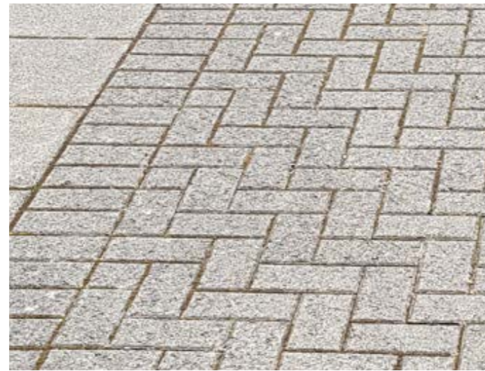
Existing block paving around City Hall
