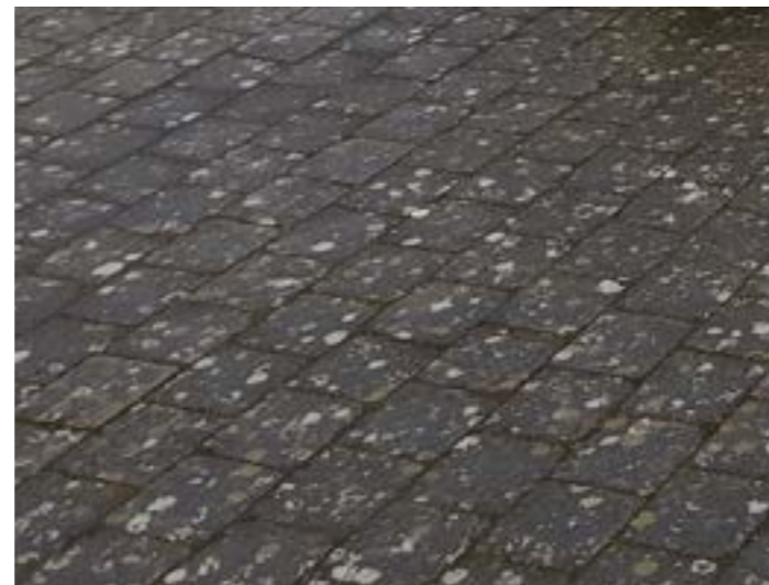
Existing sett paving around Courthouse and associated quay
