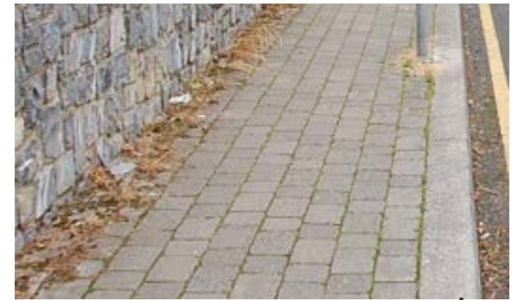
Existing block paving around City Hall
