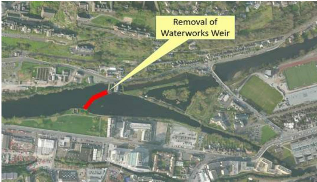
Figure 45: Removal of Waterworks Weir
