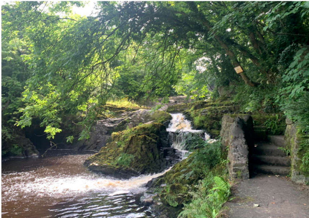
Weir located on the Mill watercourse in Buncrana – example of intricate steep structure
