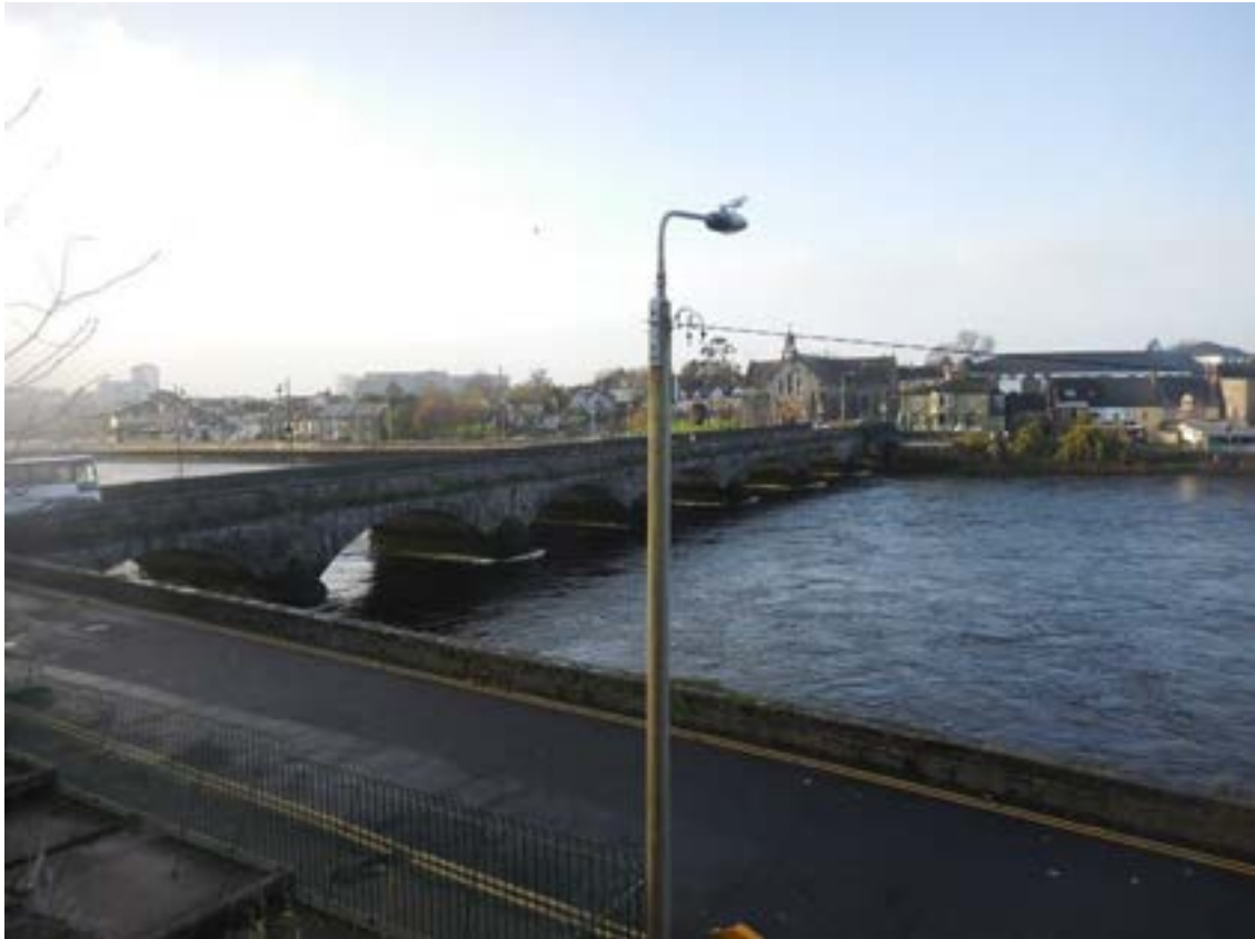
Figure 9-1. Thomond Bridge (RMP LI005-01002)
