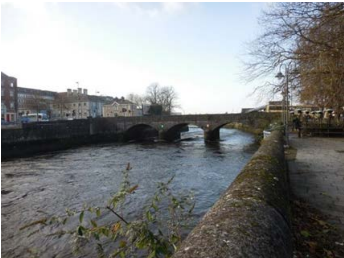
Figure 9-6. Looking West to Mathew Bridge
