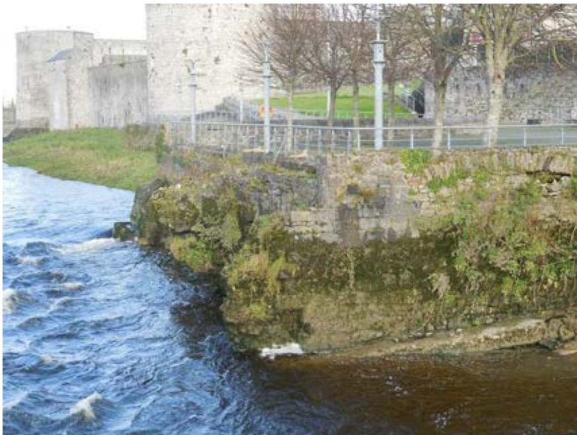
Figure 9-4. Former Site of Mill (RMP LI005-017075) near Civic Buildings
