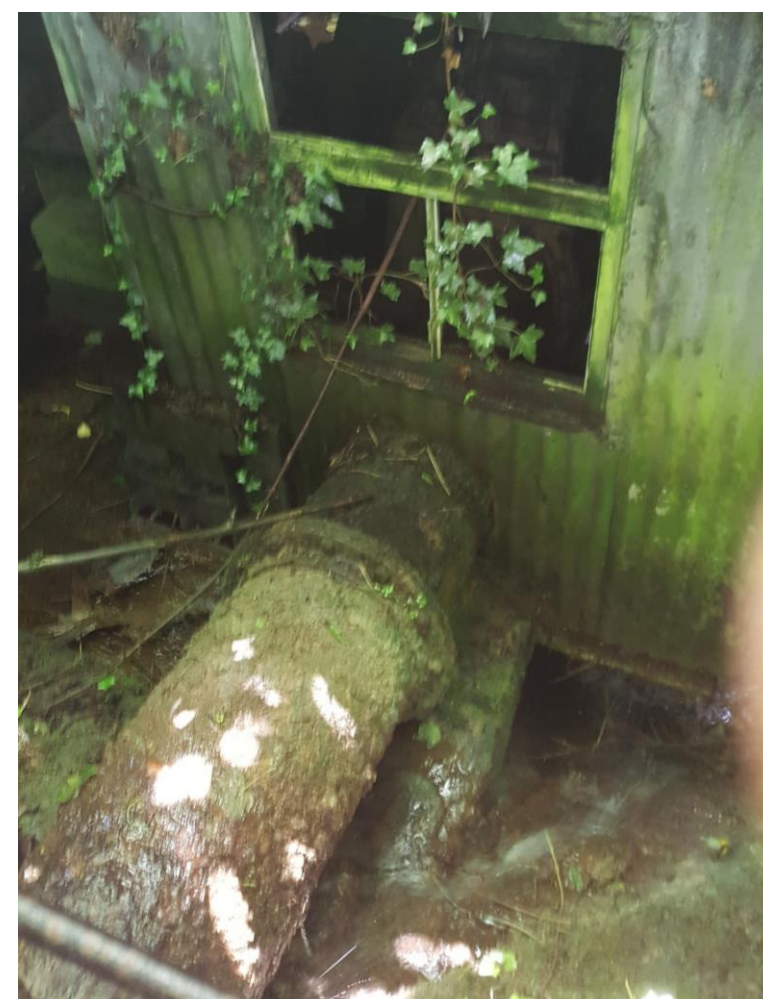
Existing sluice outlet pipe 2017
