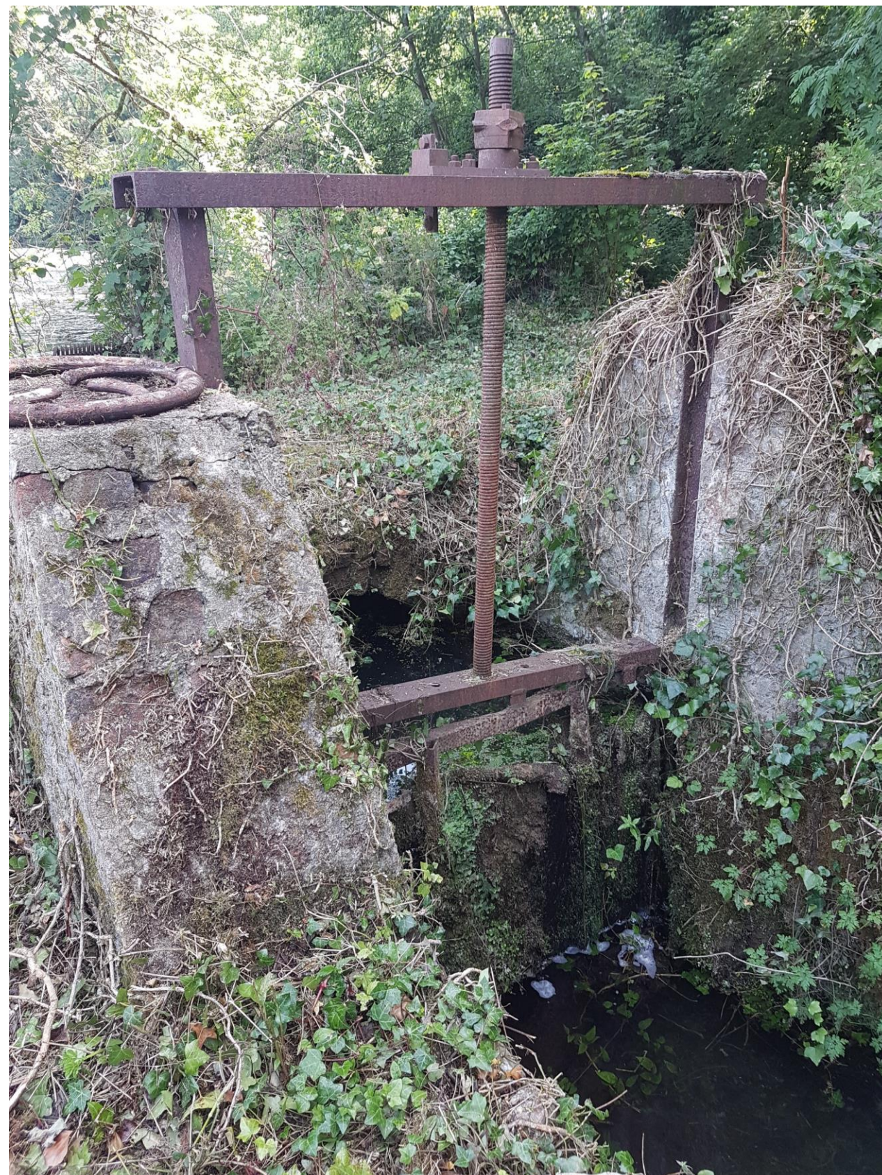
Sluice in 2017 – Looking Upstream
