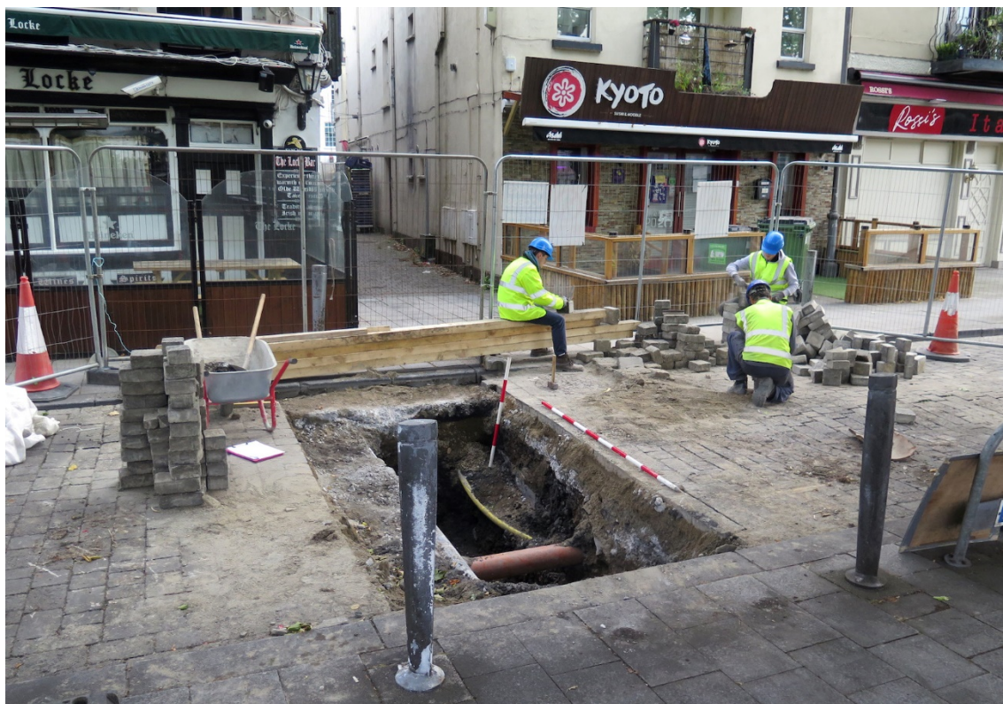
Figure 159 Location of TT7-2, facing north towards Little Creagh Lane
