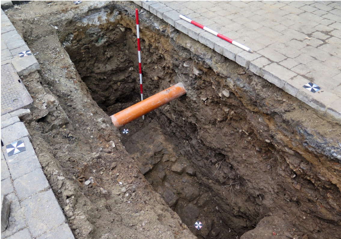
Figure 153 Northeast-facing view of TT7-1 at the completion of excavation
