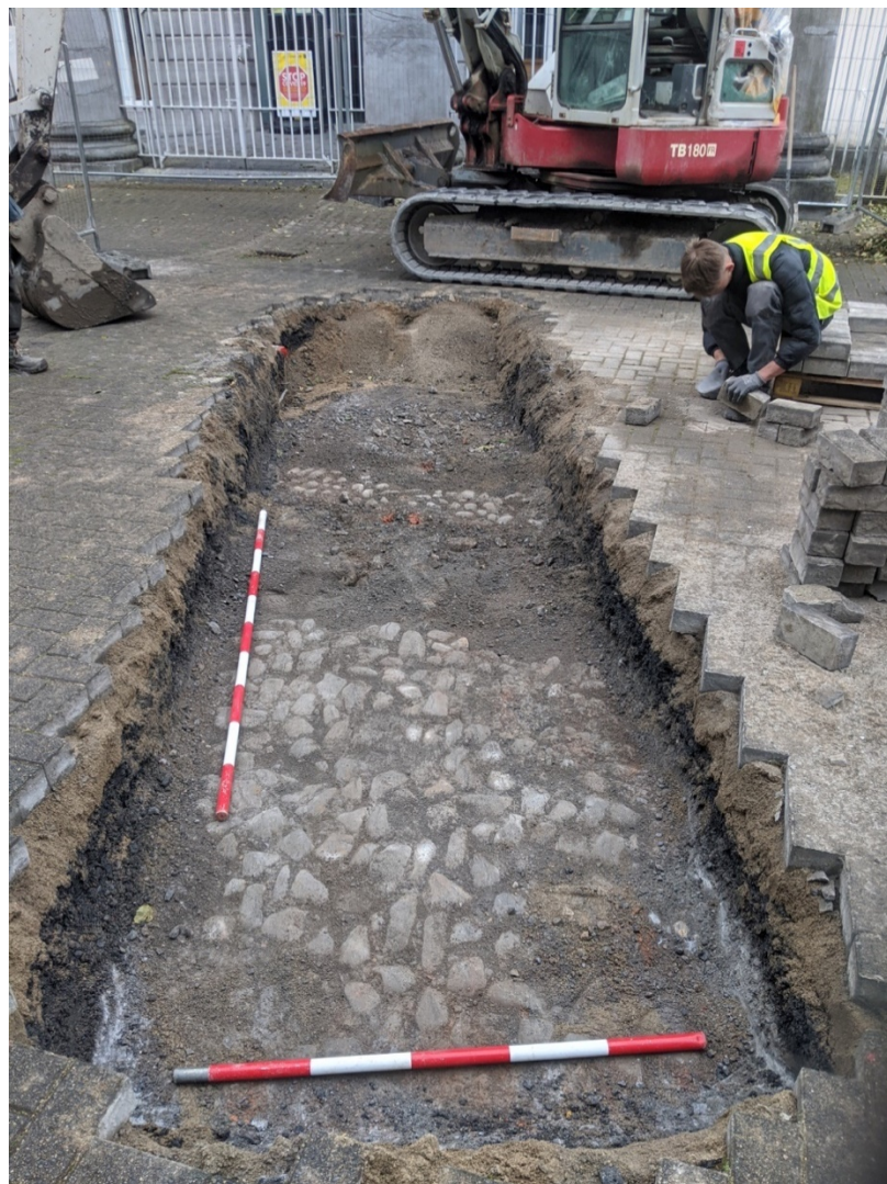
Figure 148 Cobbled surface outside Courthouse in TT6-5.
