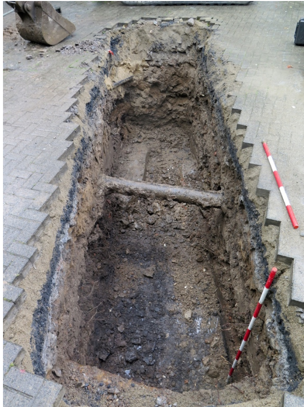
Figure 149 Depth of excavation TT6-5, showing cast pipe service.
