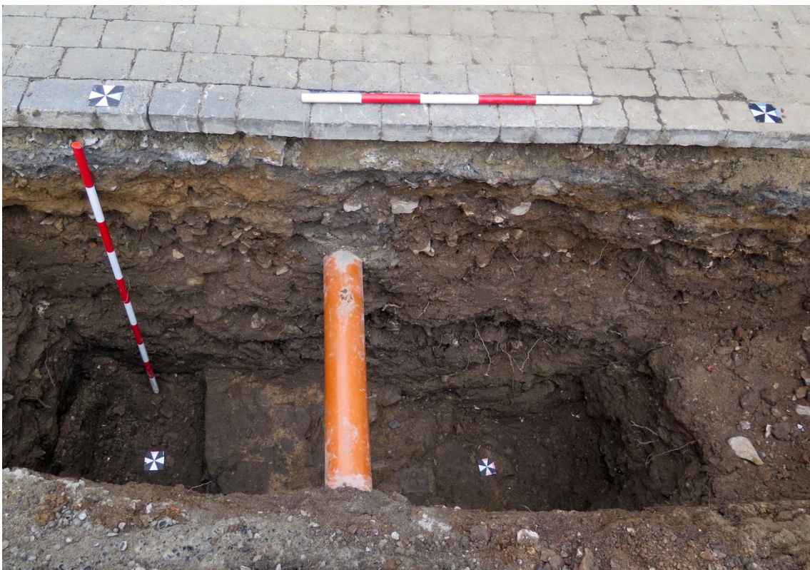
Figure 154 West-facing profile of TT7-1 at the completion of excavation
