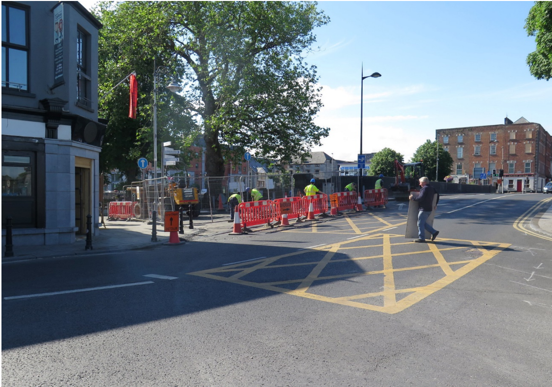
Figure 151 Location of TT7-1, facing south towards Matthew Bridge
