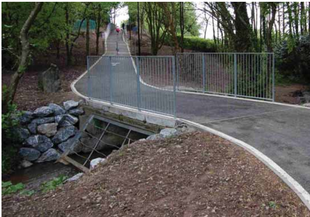
Figure 13: Existing roughing screen at Ballybrack Woods
