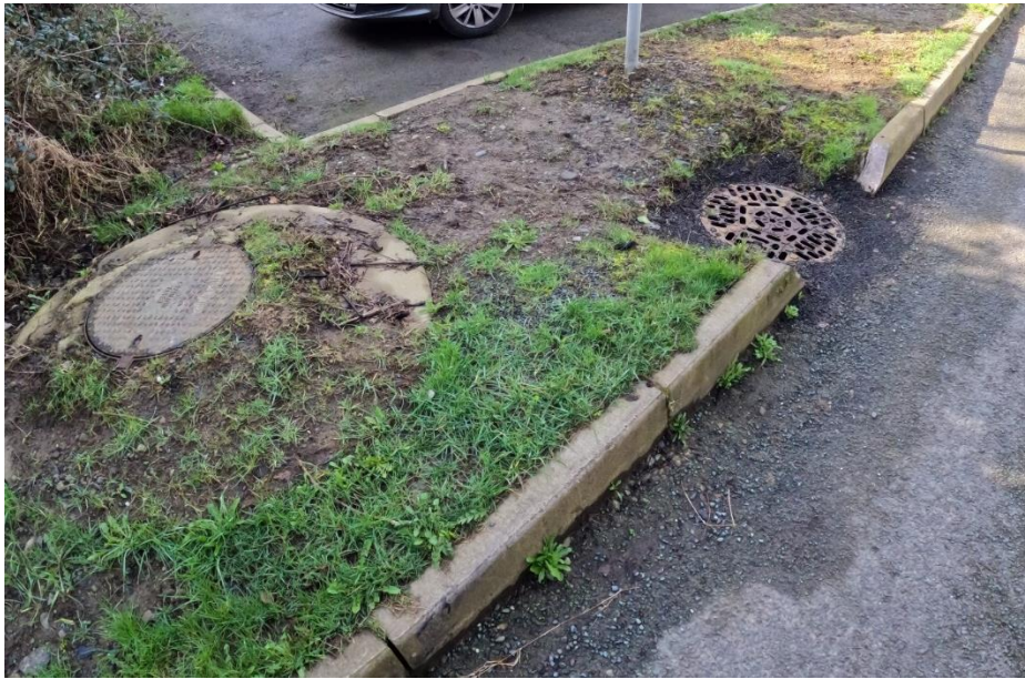
Figure 2-7 - Utility provision at The Maples housing estate
