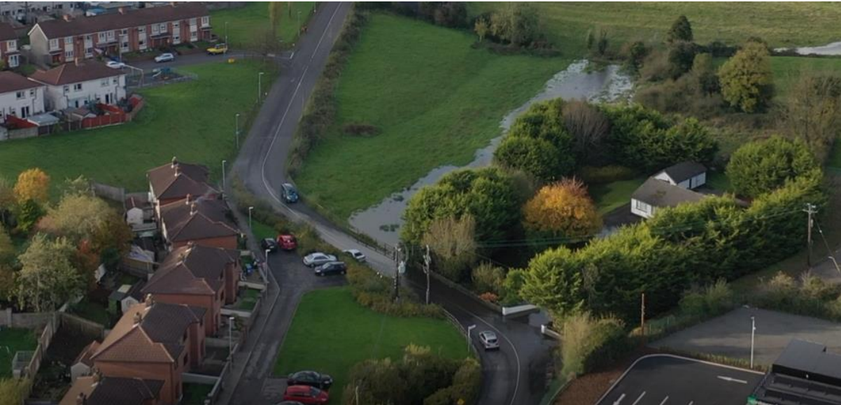
Figure 2-22 - Drone footage indicating flooded road near Laragh Crescent from route of Dublin Road to Tullymongan - Extract 2
