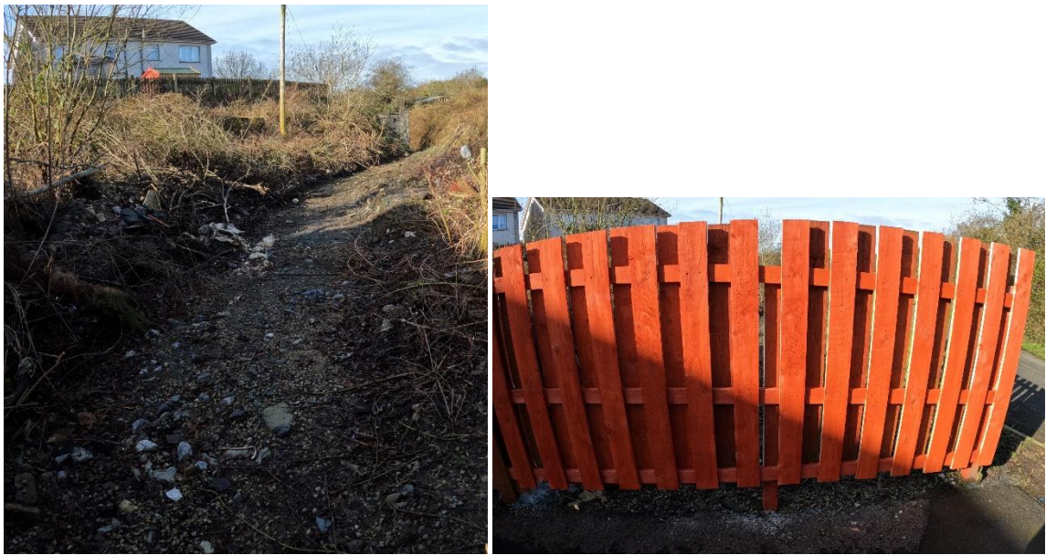
Figure 2-8 - Relief route for excess water during October flood event at The Maples
