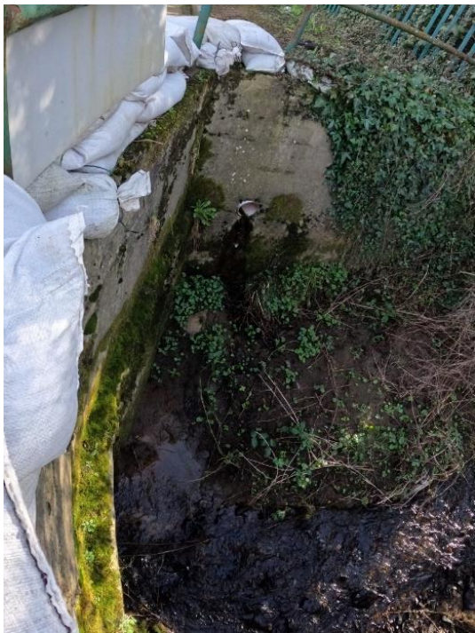
Figure 2-14 - Watercourse and culvert opening at rear of Service Station
