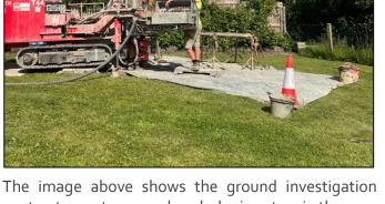
The image above shows the ground investigation contractors rotary core borehole rig set up in the near the River Finnihy in June 2024.
