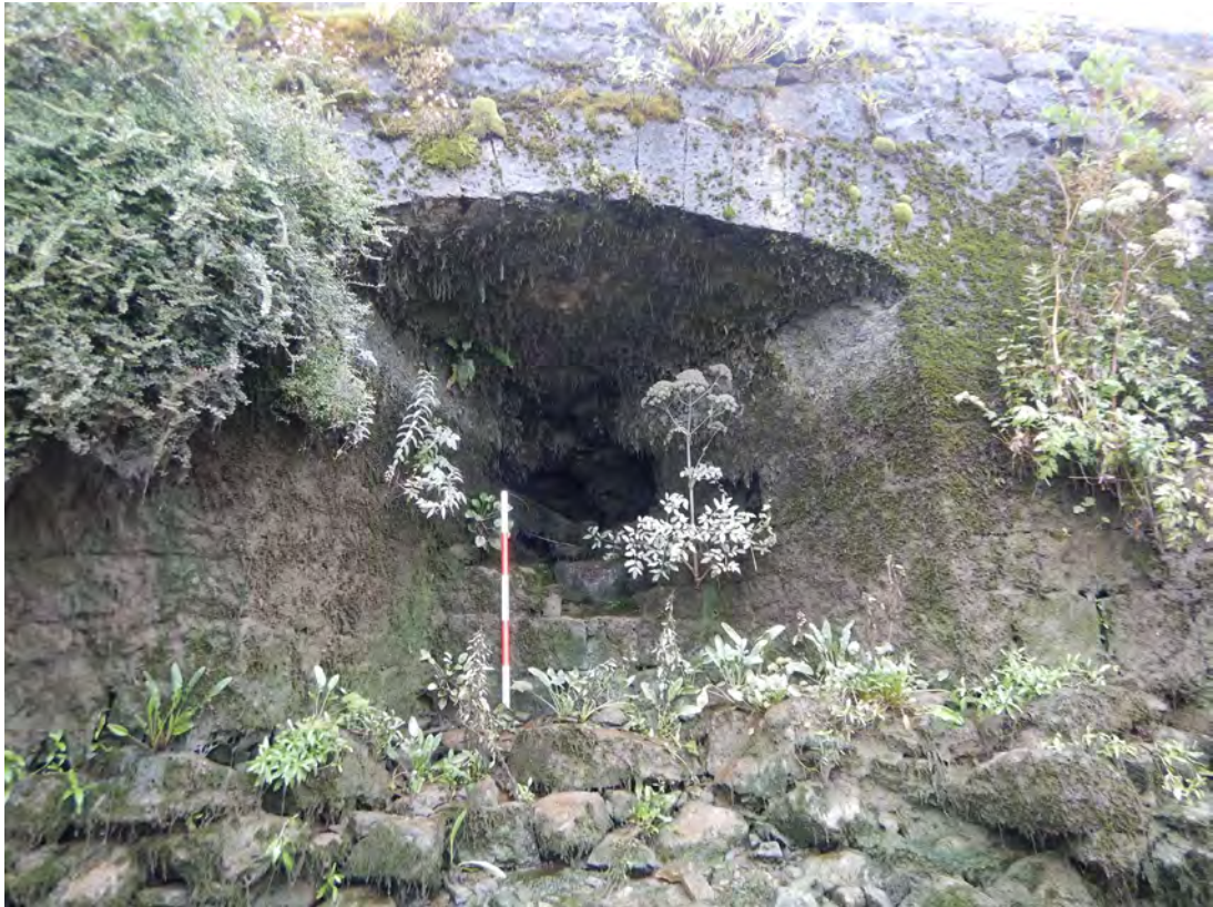
Plate 16 Archway in quay wall, taken from west.
