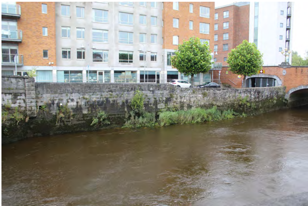
Plate 8 Quay wall between Baal's Bridge and Abbey Bridge, showing two distinct construction styles. Taken from south.
