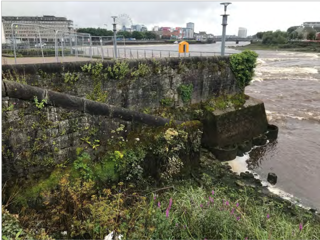
Plate 14 Access stairs and concrete cutwater, taken from northeast.
