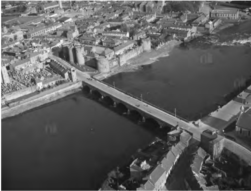
Plate 5 Thomond Bridge and King John's Castle, Limerick City, Co. Limerick by Alexander Campbell Morgan, April 1956 (NLI). Note the buildings immediately atop the quay wall to the south (right) of the King John's Castle.
