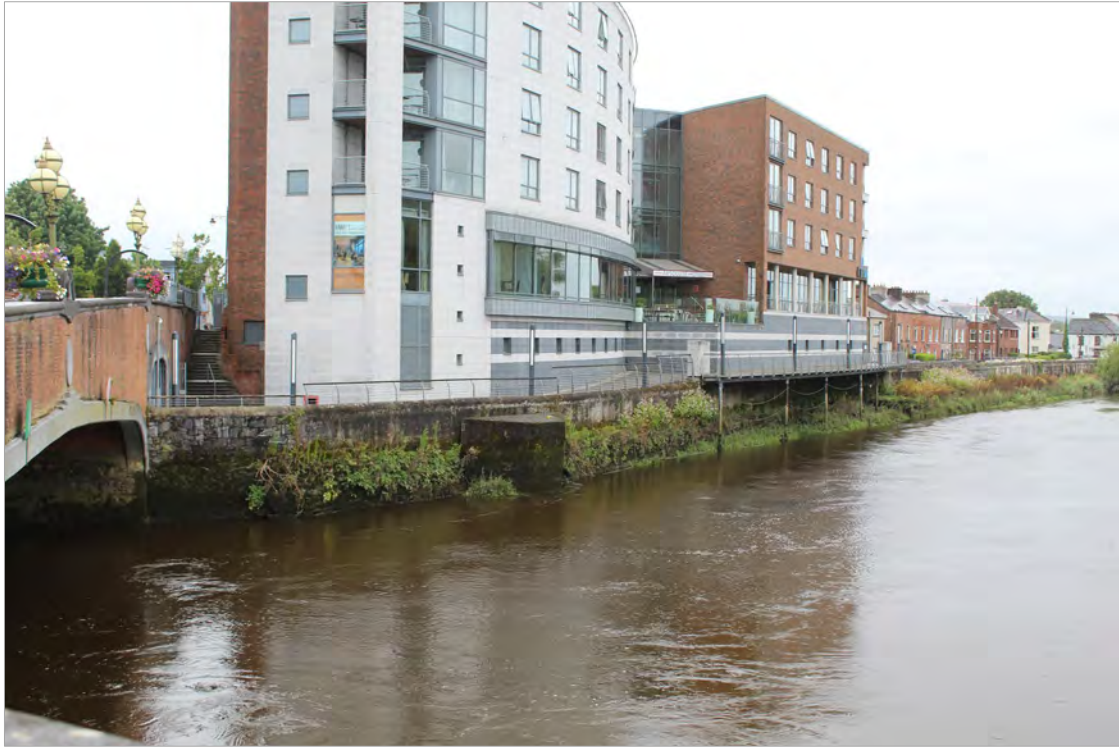
Plate 9 View from Abbey Bridge to the boardwalk, taken from south.
