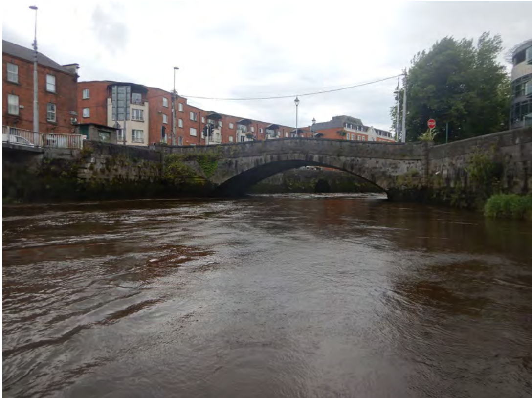
Plate 7 Baal's Bridge taken from east.
