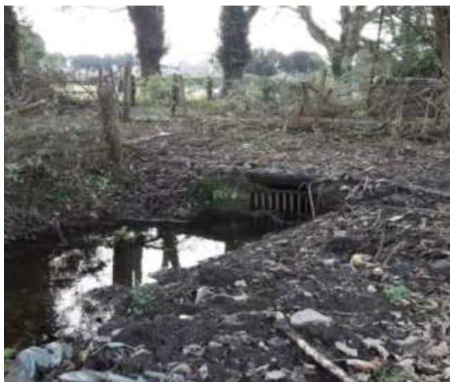
Figure 7 Trashscreen at the entrance to the culvert which conveys Trib 14 underneath the Creagh Road
