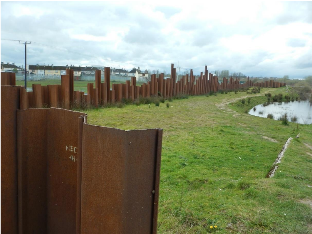
Plate 8-13: Sheet piling and earthen pathway
