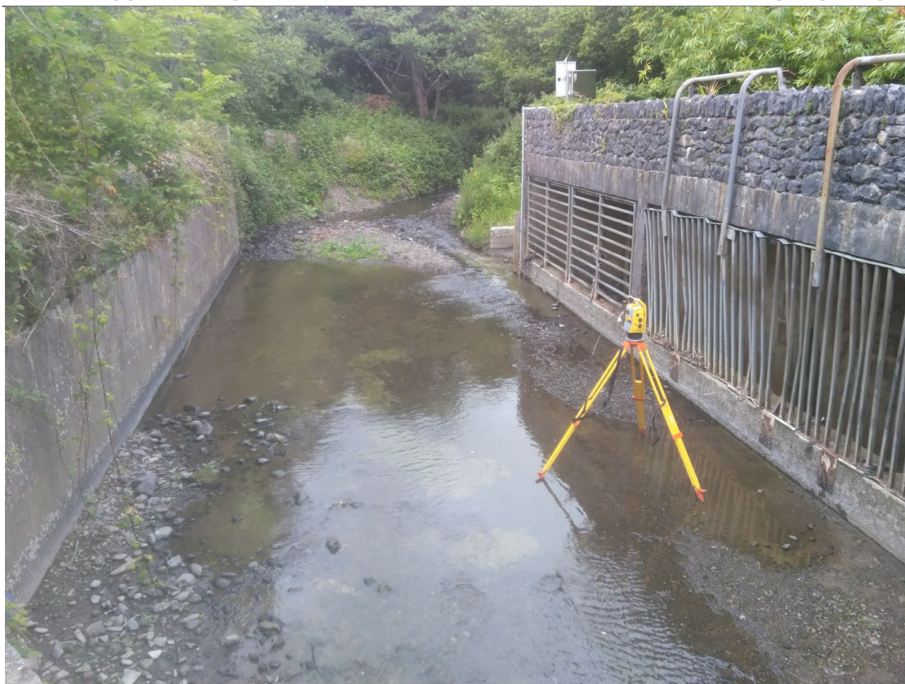
Figure 3.64: Culvert Inlet of the Big River Diversion
