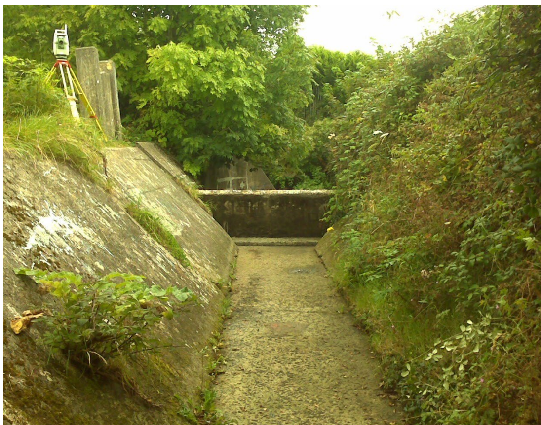
Figure 3.3: Concrete Lined Channel of the diversion between Balloonagh and Big River
