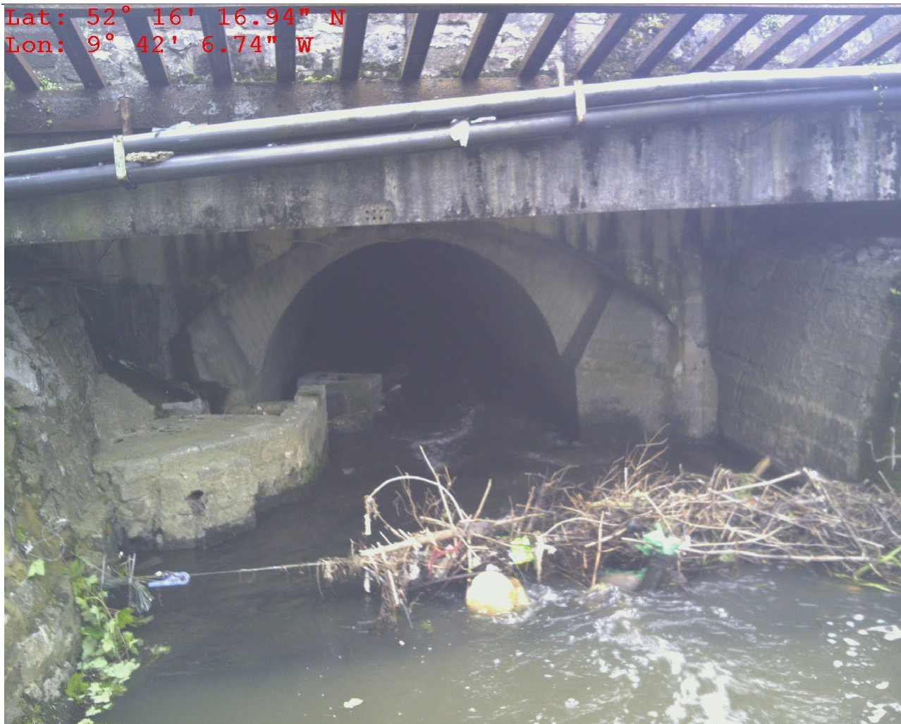
Figure 3.60: Big River Long Culvert Upstream Opening
