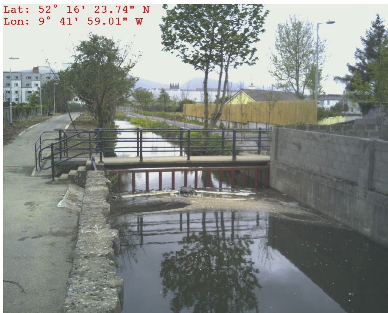
Figure 3.61: Big River Bridge and Trash Screen
