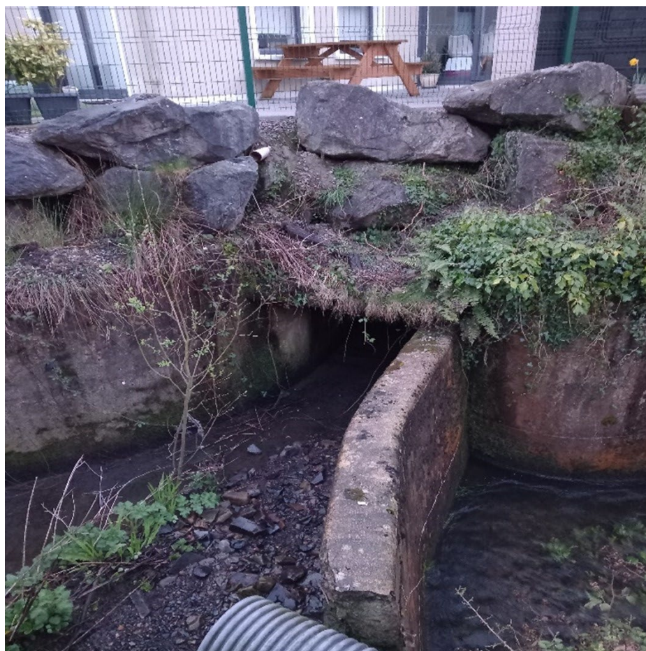
Figure 3.63: Culvert inlet of the Balloonagh to Big River Diversion
