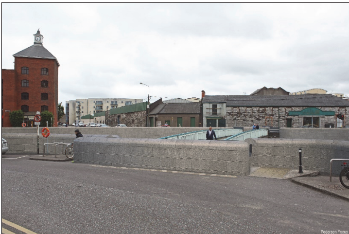
Proposed view of new flood defence walls to be closed off with flood gates when necessary
