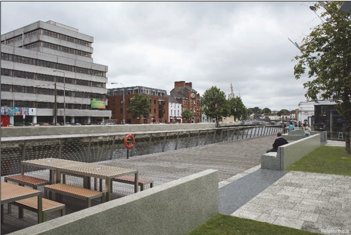
Proposed view of flood defence walls doubling as public seating with "tilt-up" or demountable flood barriers to fill gaps
