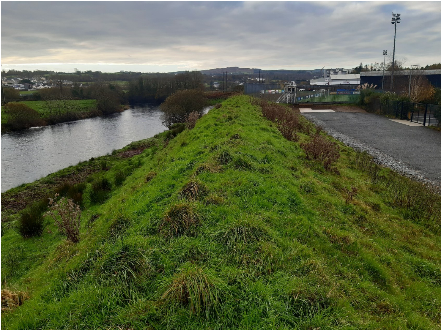
Ballybofey embankment looking towards Finn Park
