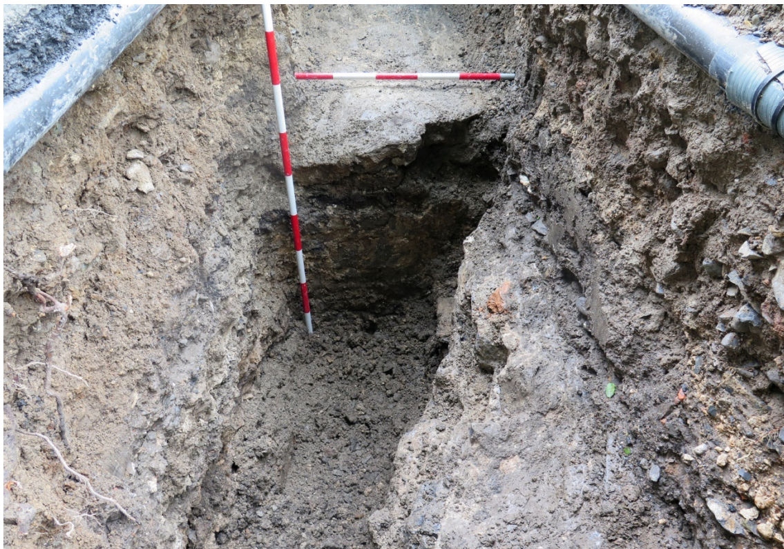
Figure 123 Looking north to wall and foundation
