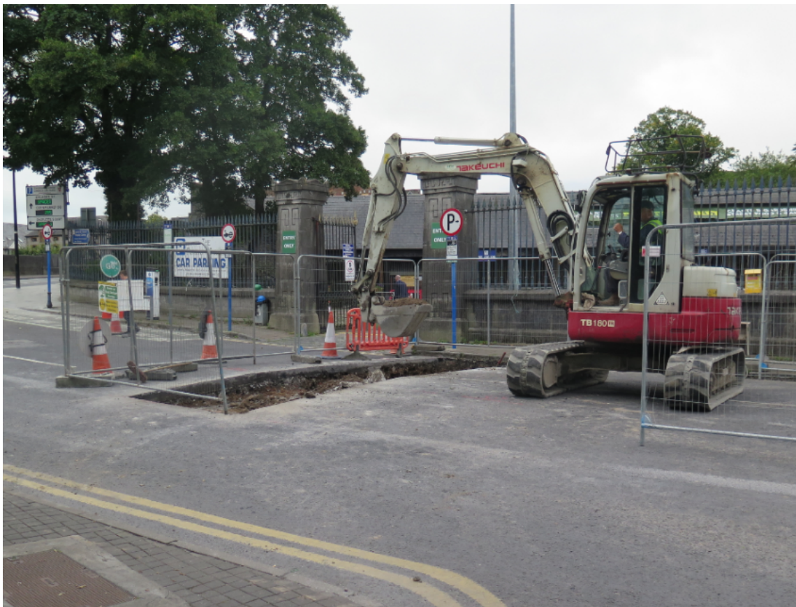
Figure 132 South-facing view of excavations in TT6-2.
