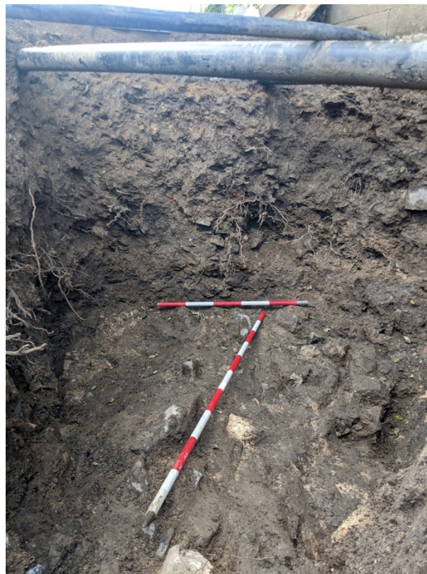
Figure 127 Southern end of TT6-1CD showing top of foundation.
