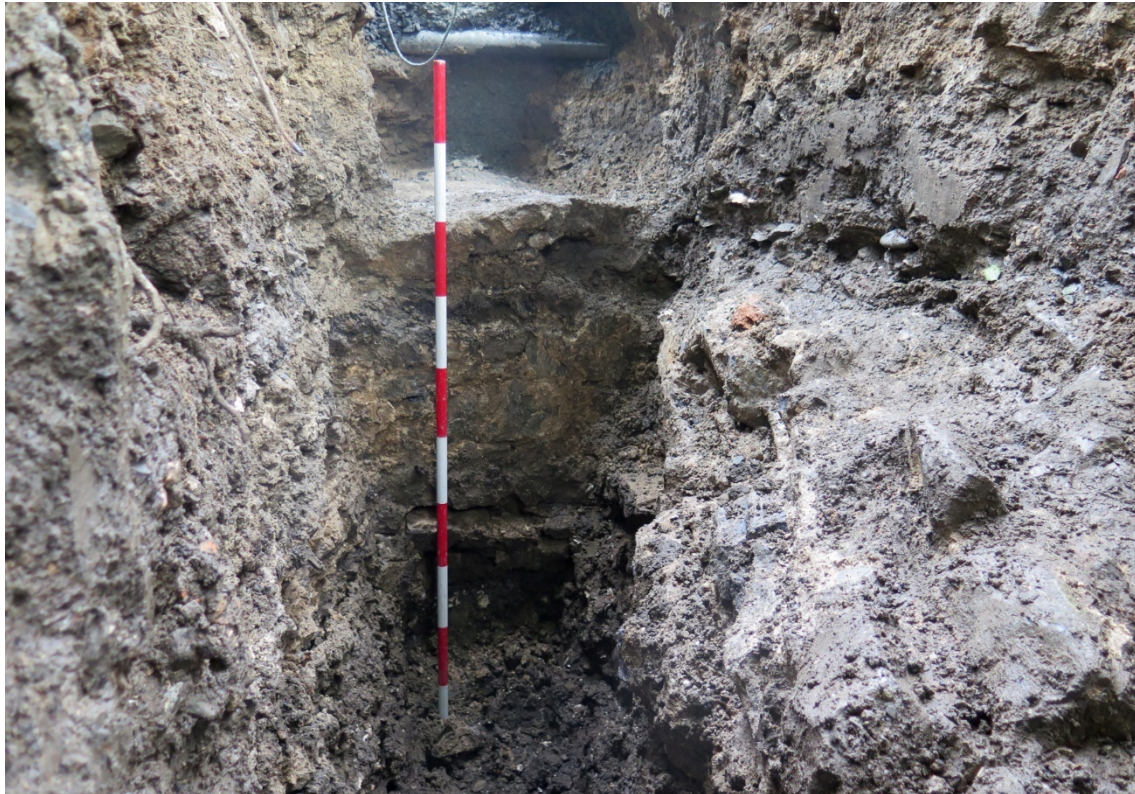
Figure 122 Northern elevation of wall and west face of foundation
