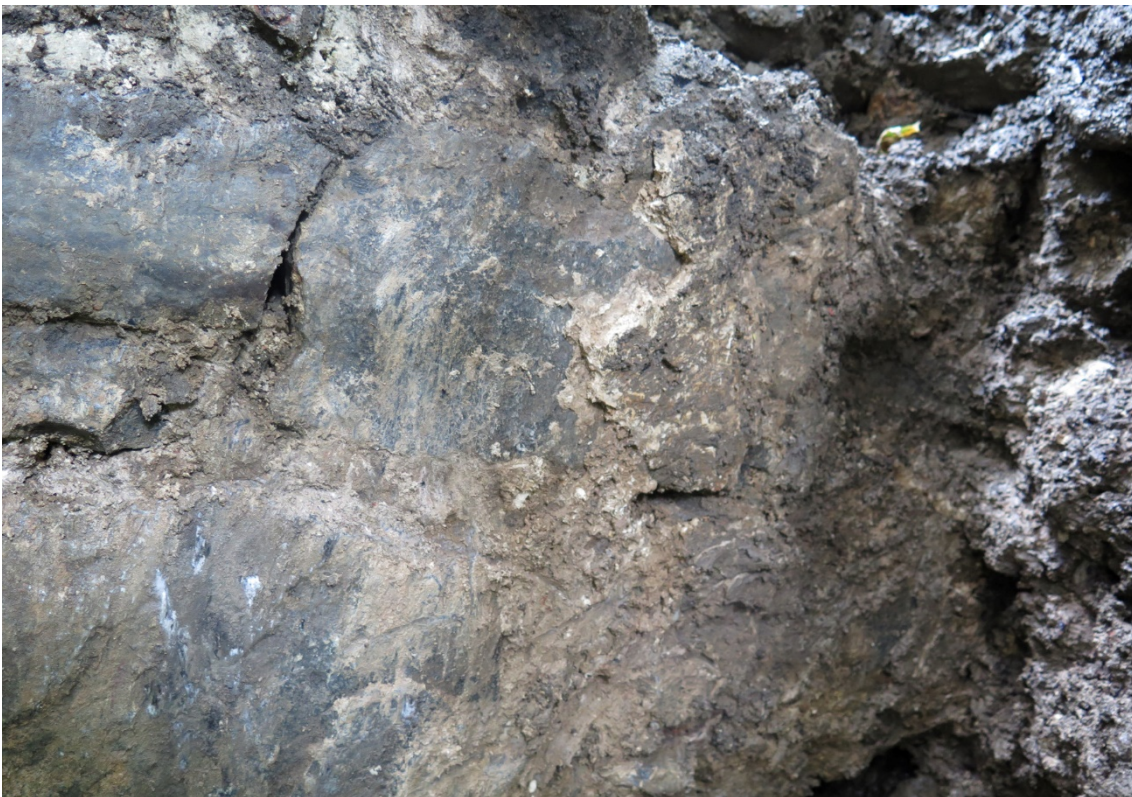
Figure 125 Evidence of render on north elevation of wall
