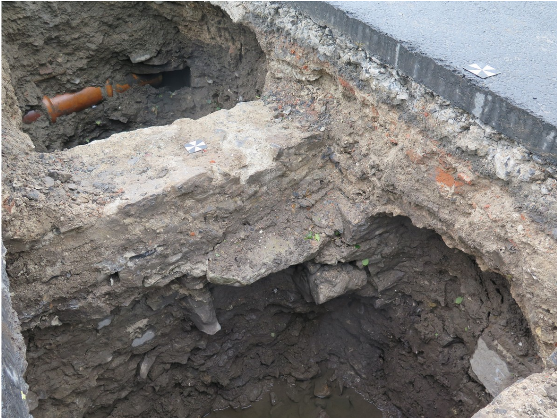
Figure 137 TT6-3, facing southwest, showing southernmost wall over box drain and lower foundation
