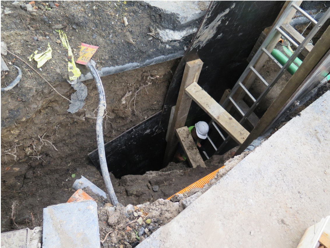
Figure 124 Deep excavation TT6-1, trench dug to a maximum depth of 4.2m
