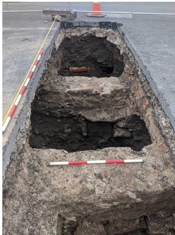
Figure 136 Southwest-facing view of TT6-3 to exposed upper foundations over a box drain.
