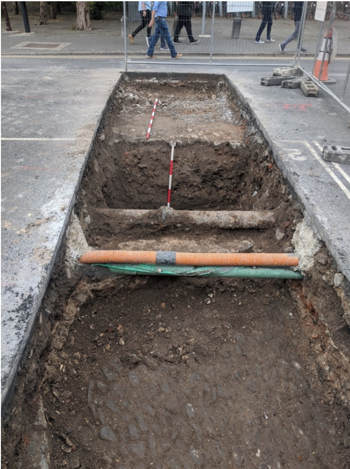
Figure 133 Two levels of cobbles and pipes over wall in TT6-2, facing northeast.
