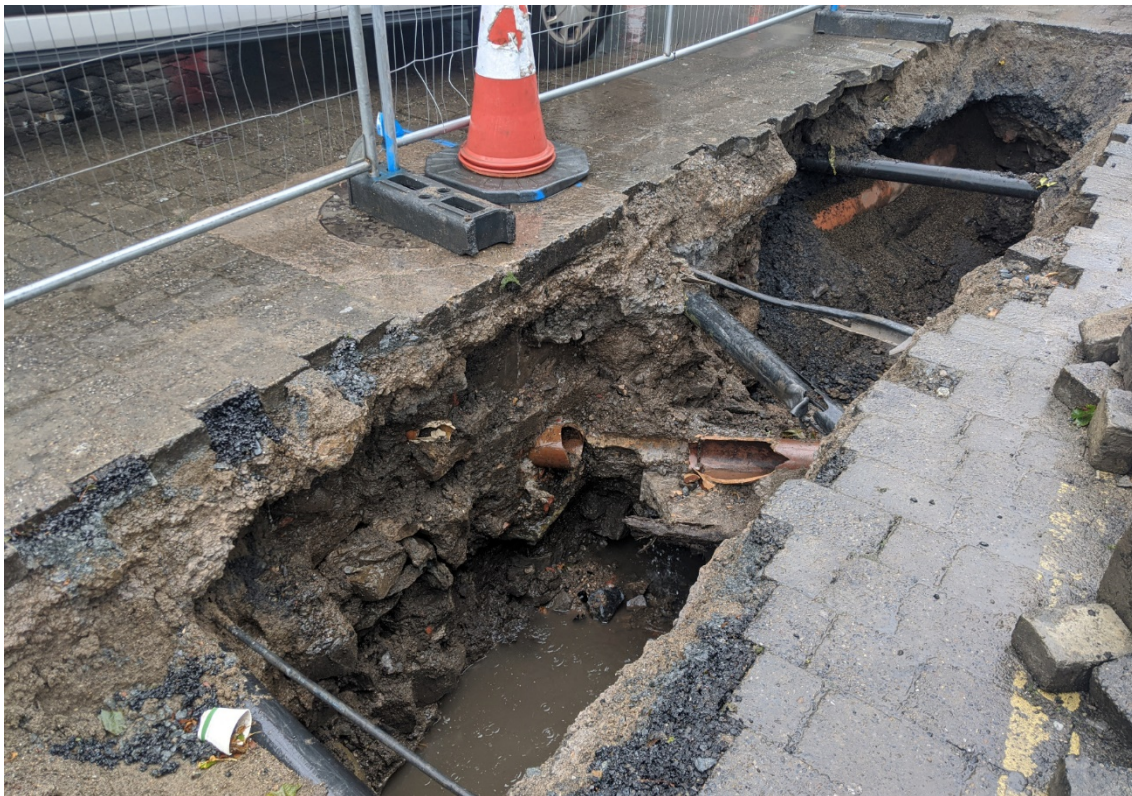
Figure 163 TT7-3 at the completion of excavation, facing north
