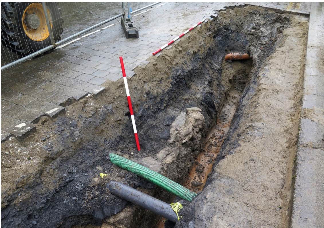
Figure 168 TT7-4, north-facing view at the completion of excavations
