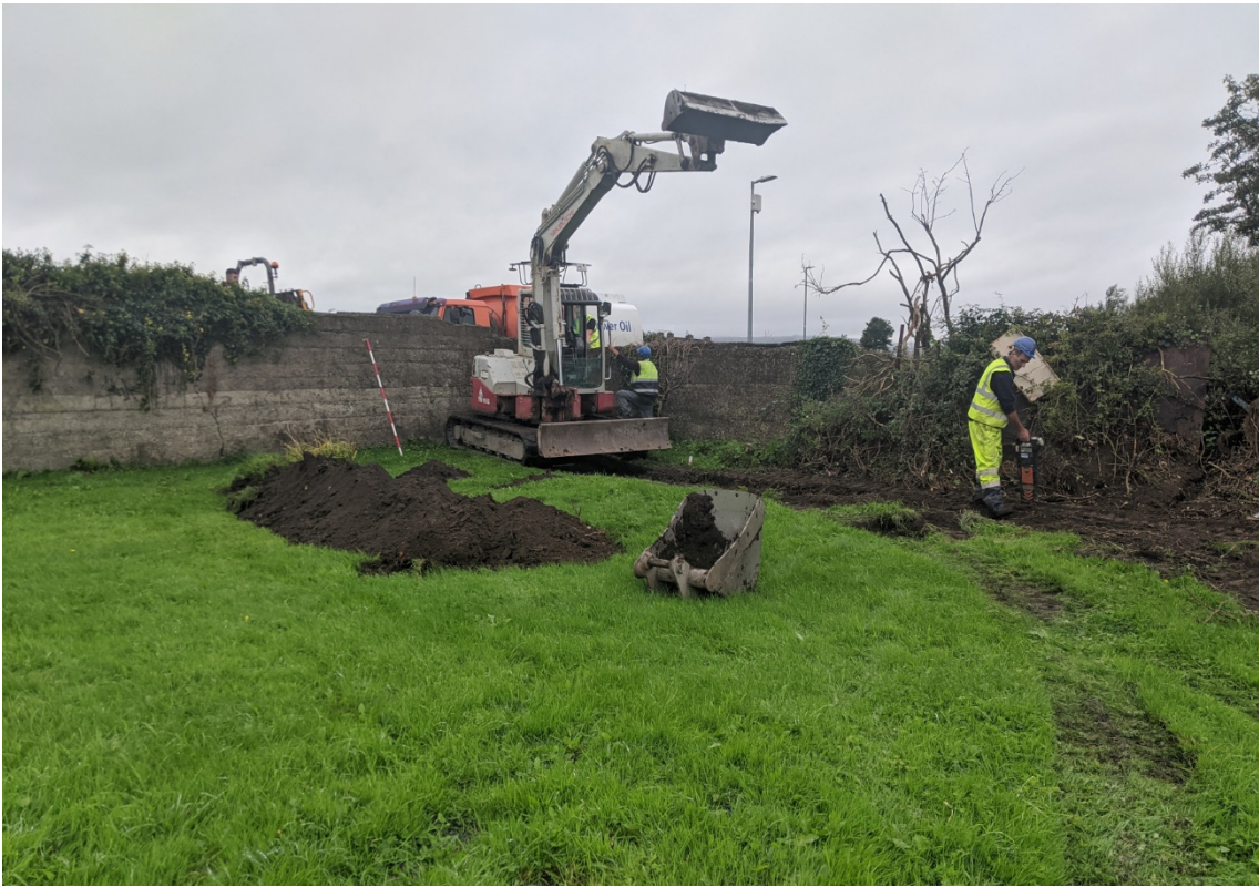
Figure 174 TT8-3, facing north near boundary wall of Athlunkard Boat Club.
