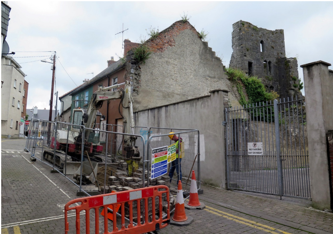
Figure 165 Location of TT7-4, facing northeast, with Fanning's Castle behind
