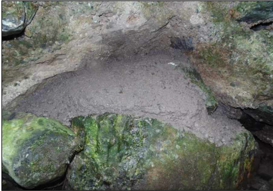
Plate 2.4 – Suspected otter holt sealed off with 30N dry concrete mix.
