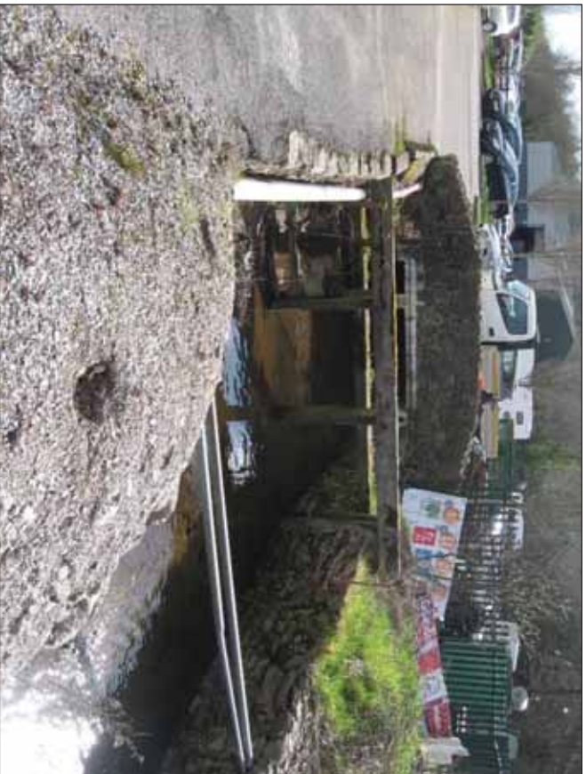
Plate 6: Mill race 3 opening in Grandon's Garage showing remains of sluice gate, before entering culvert, looking southeast
