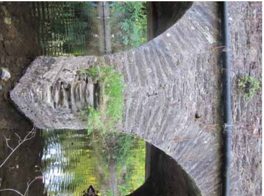
Plate 38: View of CHS 12, bridge, cutwater on downstream elevation.
