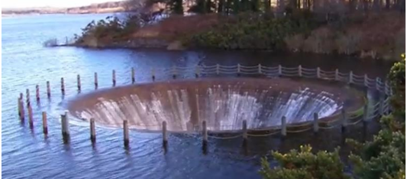
Morning Glory spillway at Varray Reservoir
