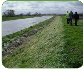
Improvement of Channel Conveyance
