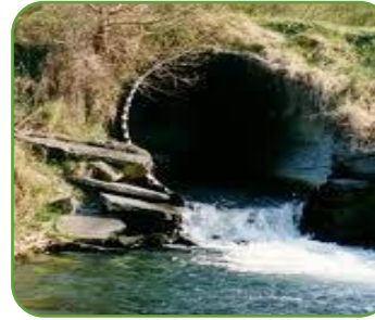
Flow diversion through culvert or open channel
