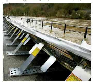
Figure 34: Typical Temporary Flood Barrier (Image: Courtesy of Geodesign AB)
