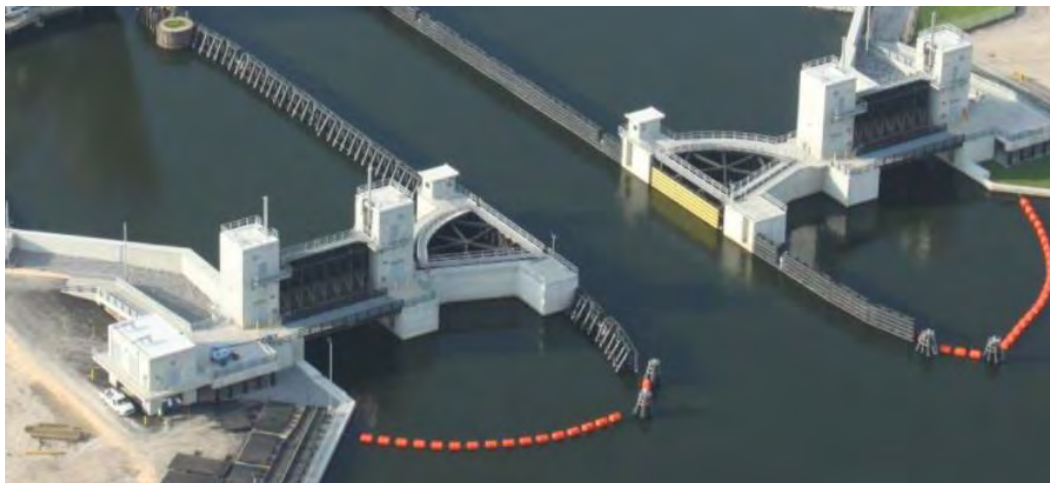
Figure 77: The Seabrook Floodgate Complex (HR Wallingford, 2017)
