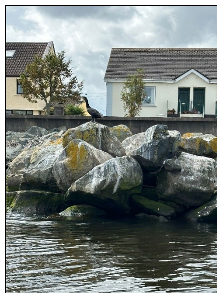
Figure 2. Bird within the scheme atop revetments.
