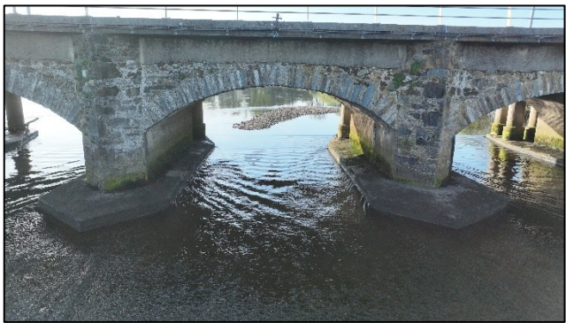
Figure 3. Drone photography of Nineteen Arch Bridge taken during condition survey.
