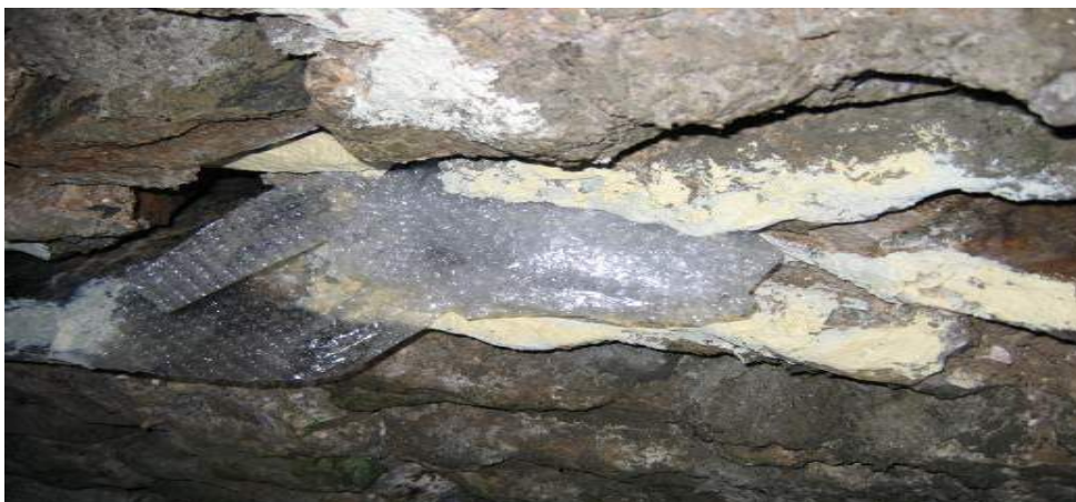
Photograph 1 Example of a bat-suitable crevice filled/blocked with bubble wrap to prevent bat occupancy during works (Photograph courtesy of Caroline Shield)
