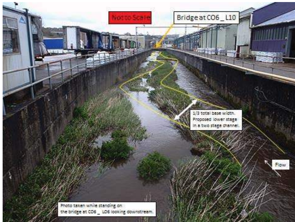
Figure 3. An outline sketch of the enhancement proposal for this reach following the implementation of the drainage programme.
