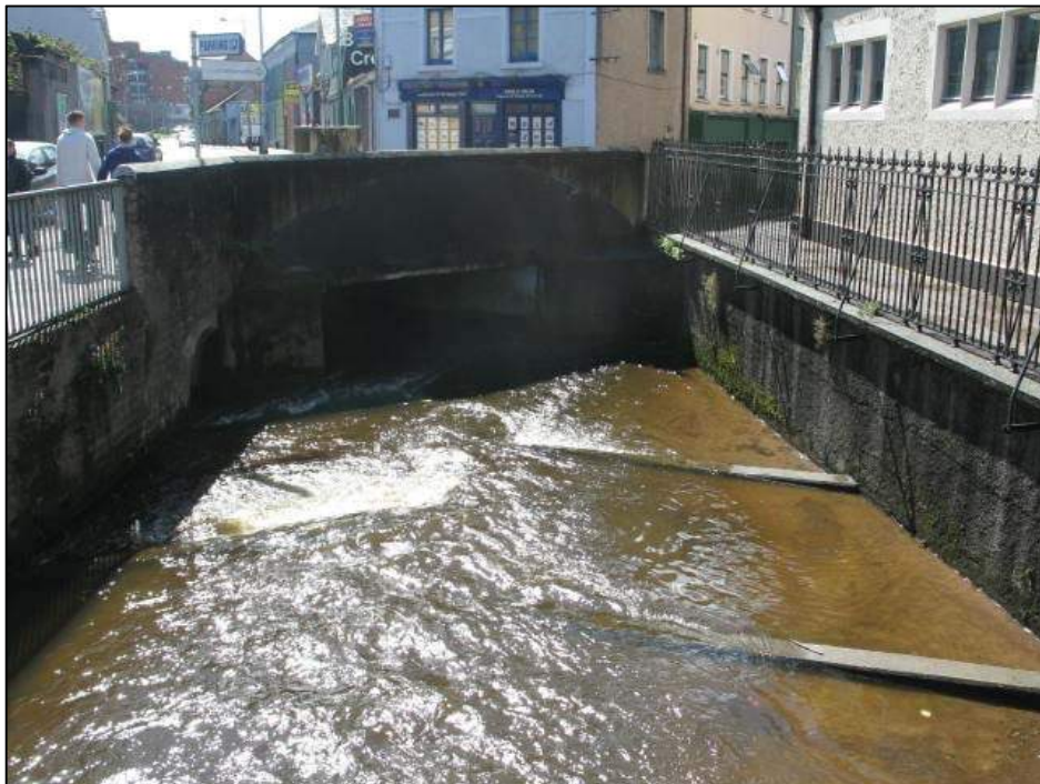
Plate 10.2: View of culvert extending under Watercourse Road from north showing concreted channel (church wall and railings visible at right)
